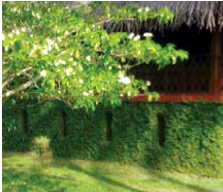
Building envelope insulation by ivy growing on walls
