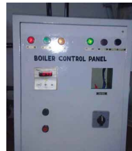
Solar thermal water boiler control panel
