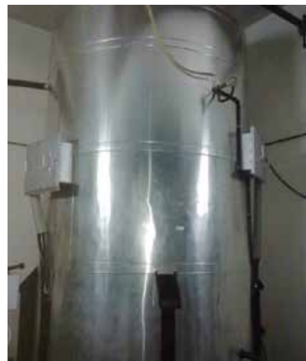
Solar thermal water storage tank
