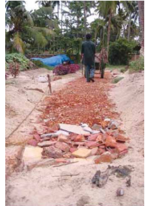
Construction debris used for pathway creation
