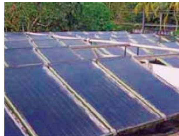
Solar Thermal panels
