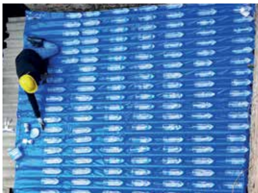
FIGURE 7: Insulation through water filled PET bottles
