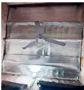
FIGURE 8: Alufoil layering under roof
