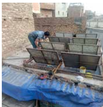
FIGURE 9: Chain-sprocket roof intervention
