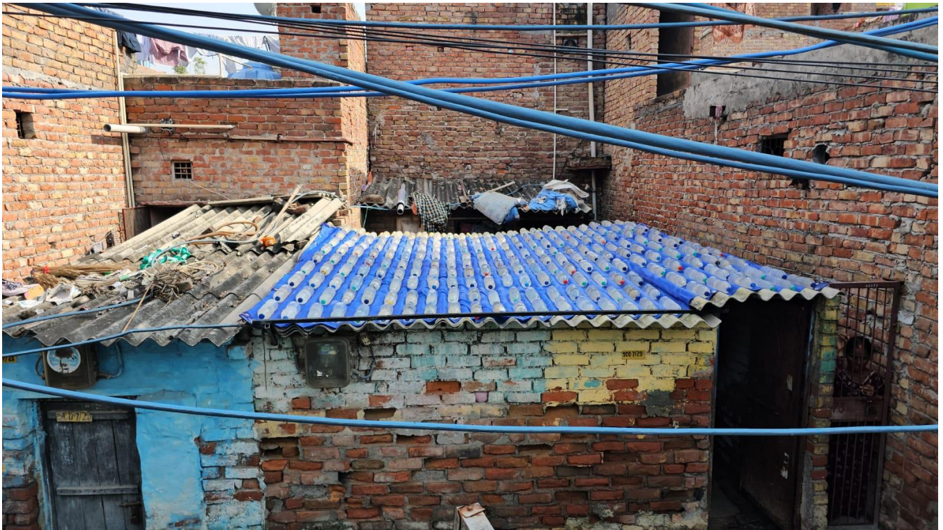
Figure 5.11: Final View After MS Strip Installation
