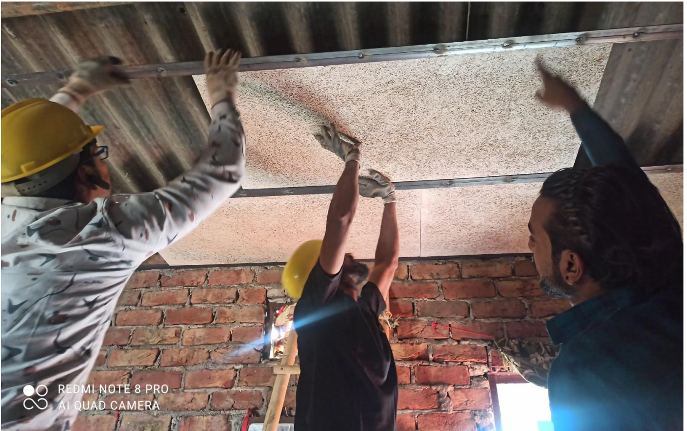
Figure 3.1: MS support frame for panels-installation in progress
