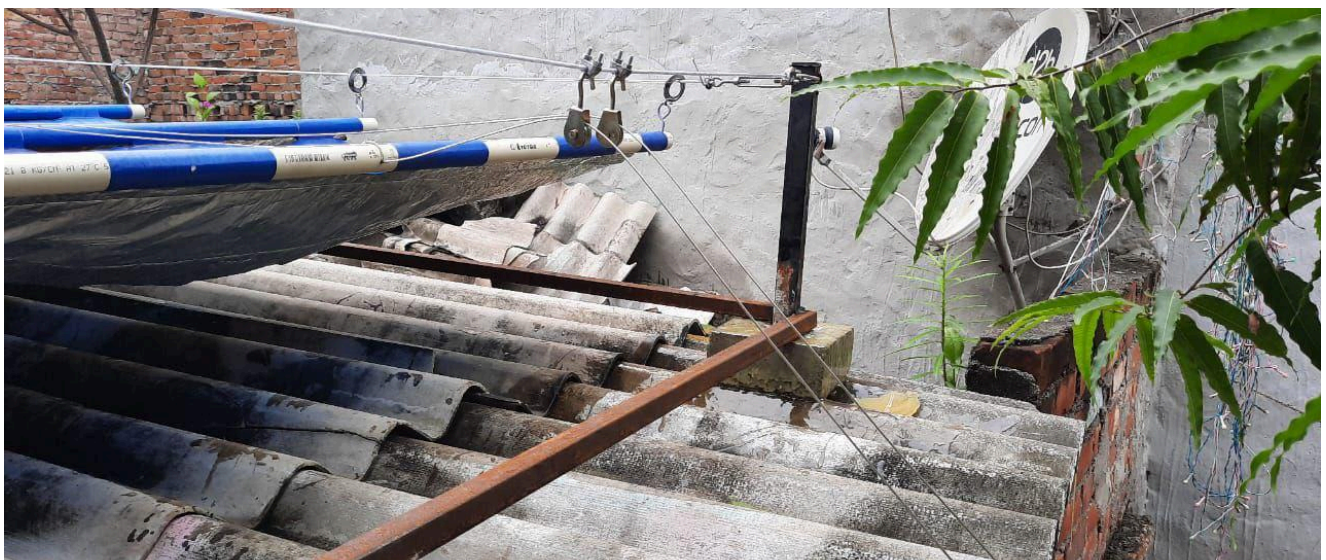
Figure 4.5 Additional Pipe Supports At The Base
