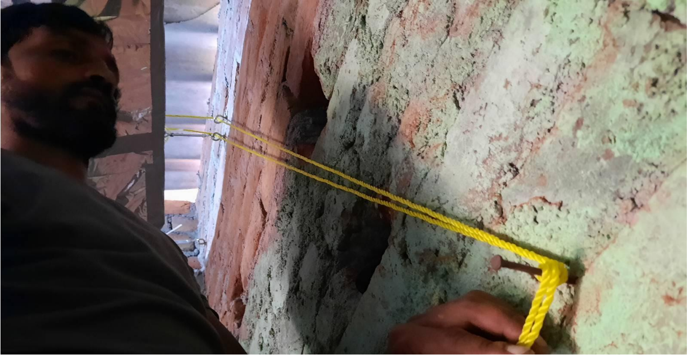
Figure 1.14: Handling mechanism at rear end - nylon wire loop going through two individual hooks.
