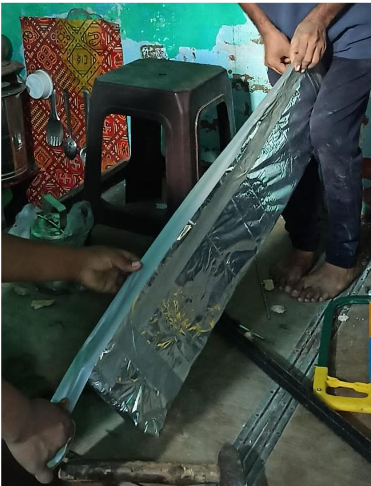
Figure 2.20: Tape the cut end with aluminium tape
