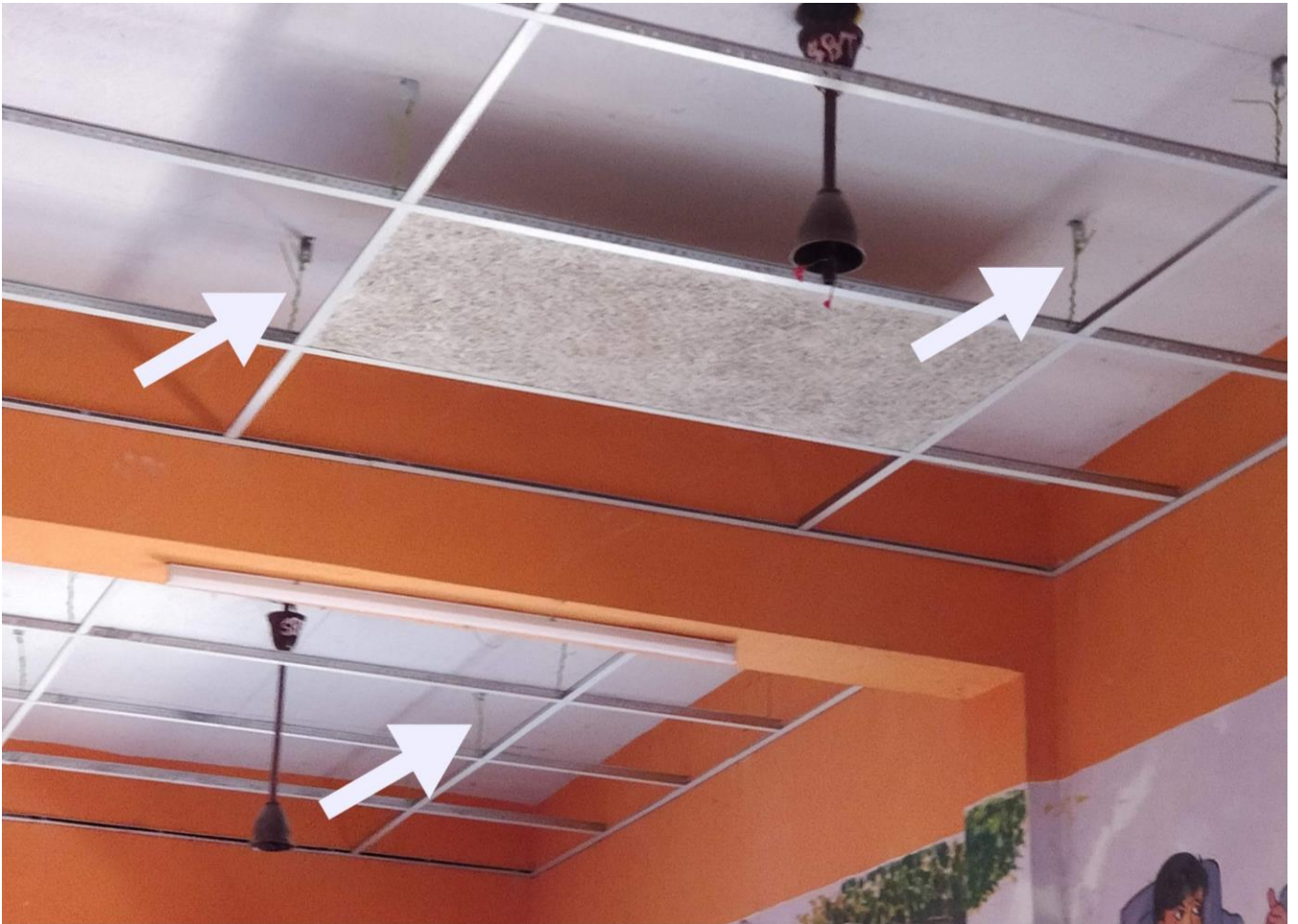
Figure 3.3: Extra roof support
