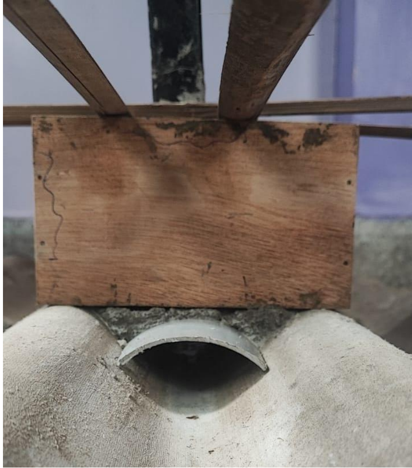
Figure 7.8: Casting the support with drip line
