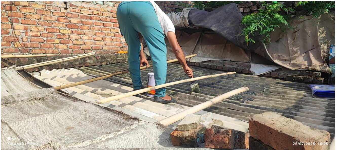
Figure 6.3: Applying Of Adhesive Above The Roof
