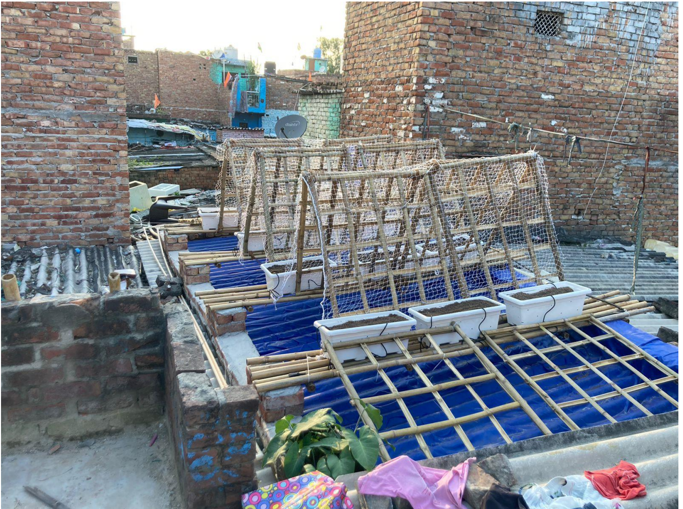
Figure 4.18.1: Rooftop Garden After Installation
