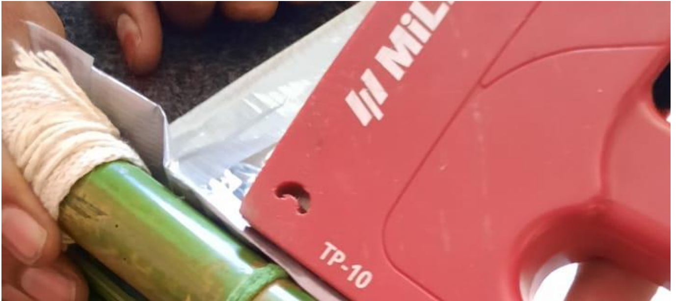
Figure 8.2: Stapling of MLP sheets on primary bamboo section
