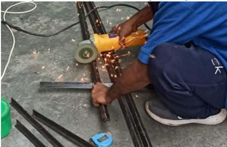
Figure 2.15: MS L-angle lengths being prepared for panel support frame
