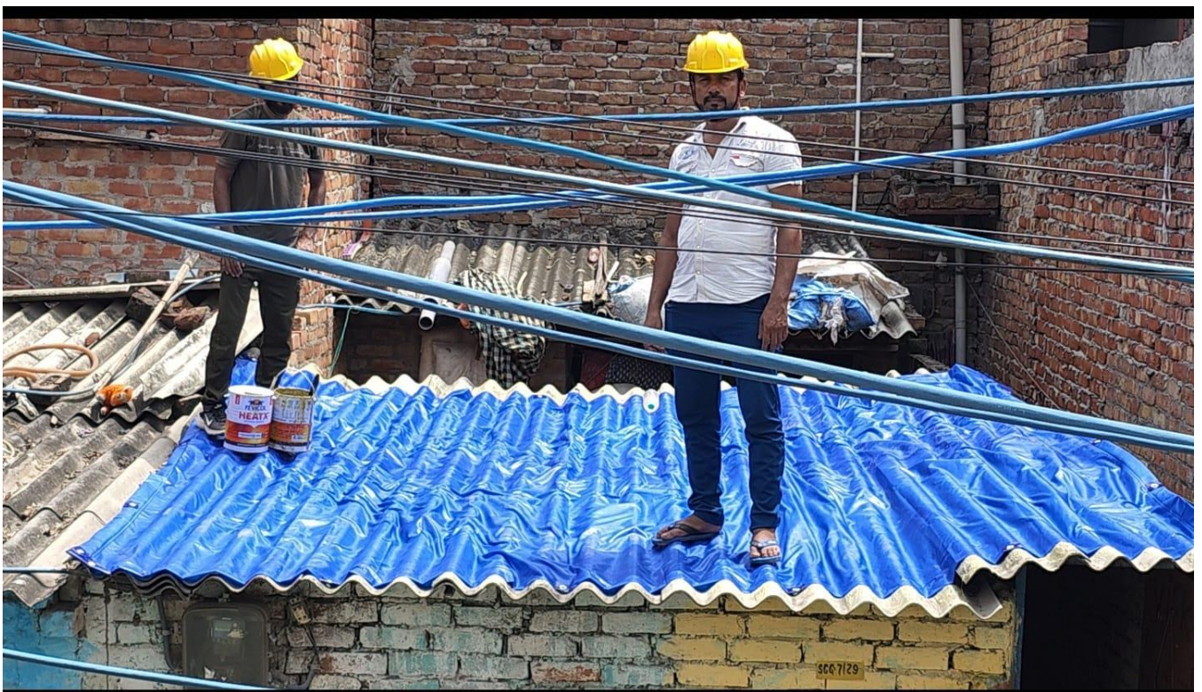
Figure 5.6: Final View After Application Of Silpaulin
