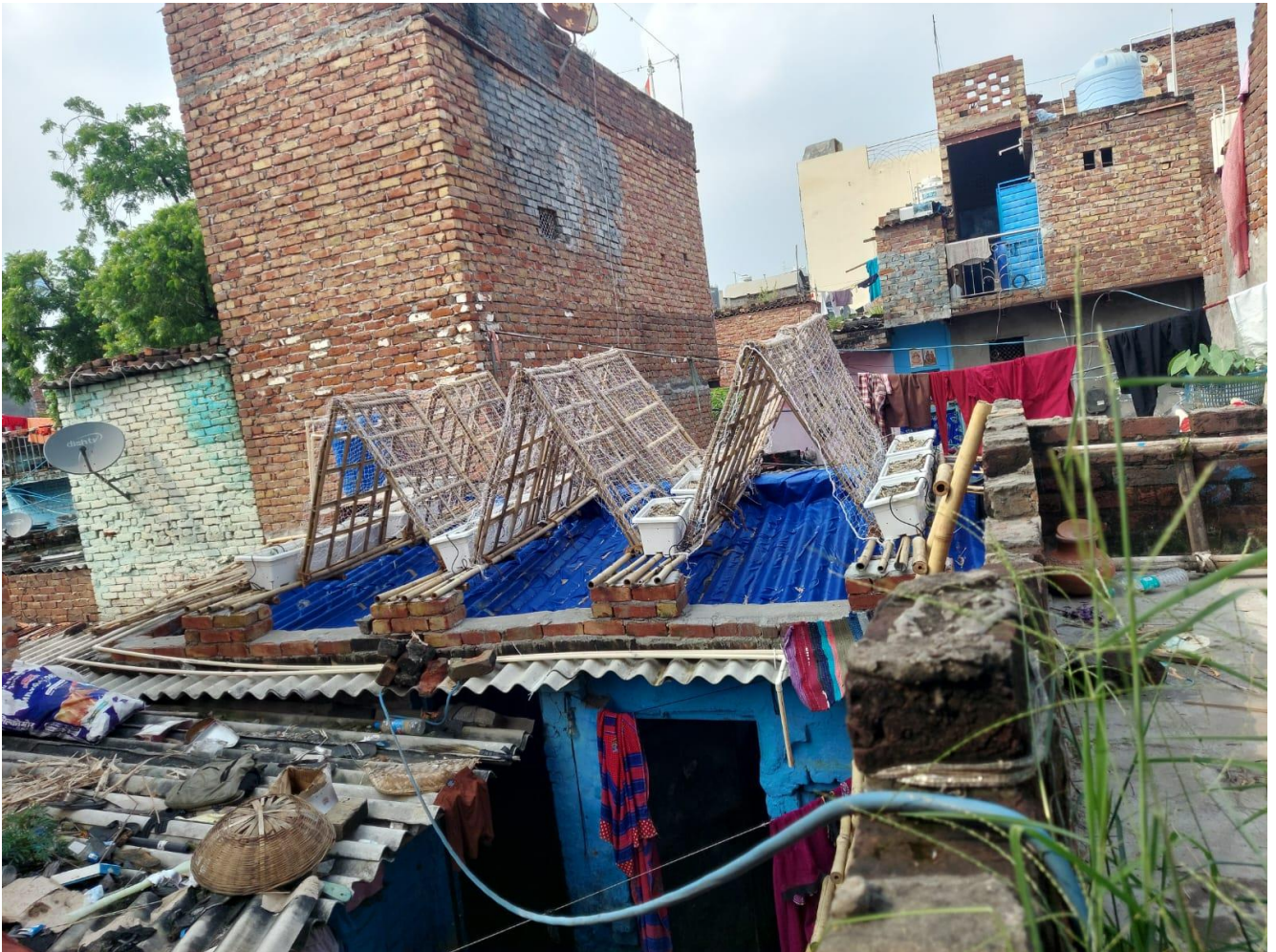
Figure 4.18.2: Rooftop Garden After Installation
