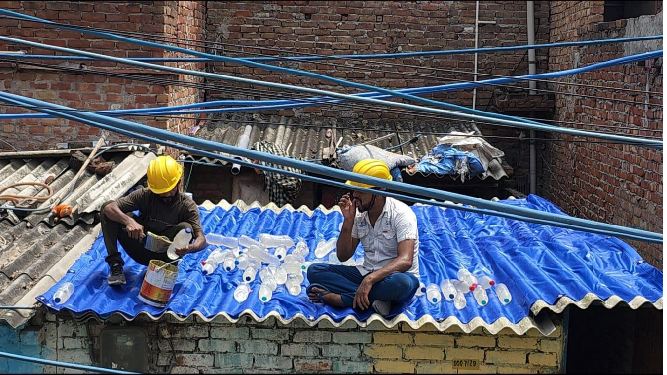
Fig 5.7: Application Of Adhesive Along The Bottle Side Which Touches The Roof
