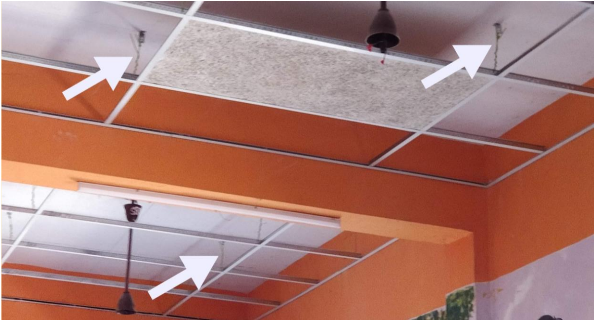
Figure 2.18: Extra roof support
