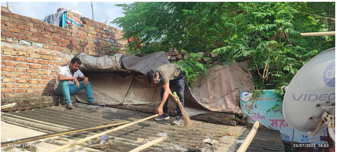
Figure 6.1: Cleaning Of Roof
