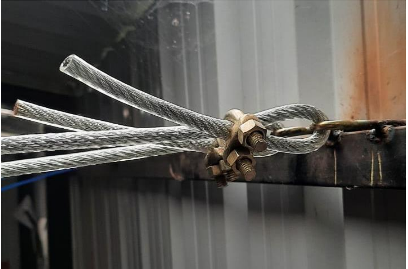
Figure 1.3: Establishing wire rope to wall using U-clamps
