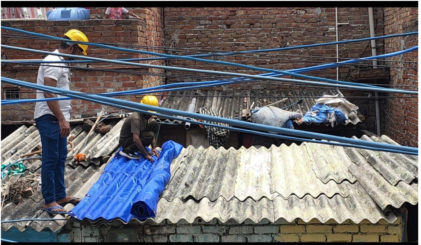
Fig 5.5: Sticking Of Silpaulin Across The Roof
