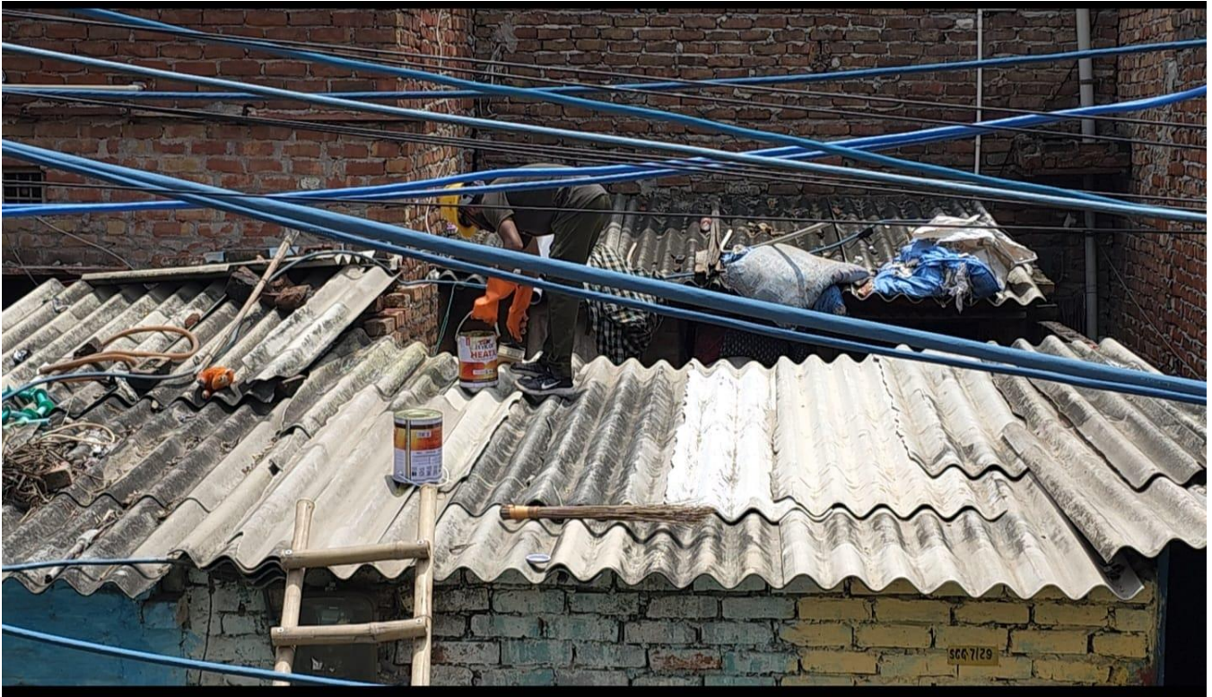
Figure 5.4: Applying Of Adhesive Over The Roof
