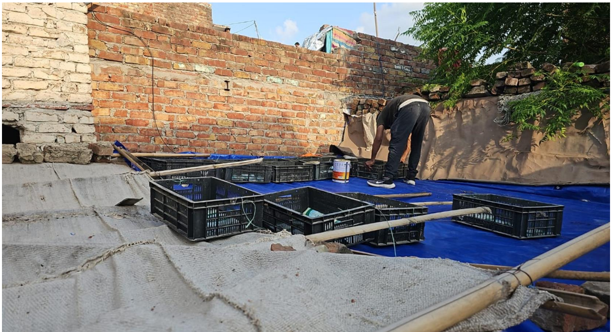
Figure 6.5: Placing Of Crates Above Roof
