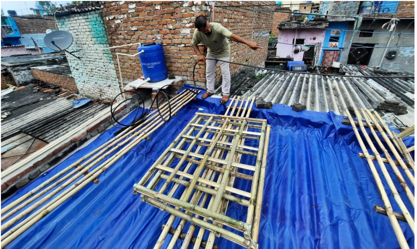
Figure 4.8: Stretching of Irrigation Hose for Installation
