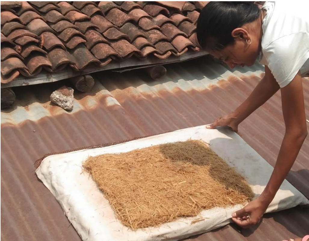
Figure 2.12: Sun-dry the panels
