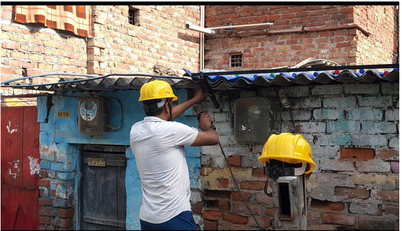
Figure 5.10: Securing Of MS Strip Through Welding
