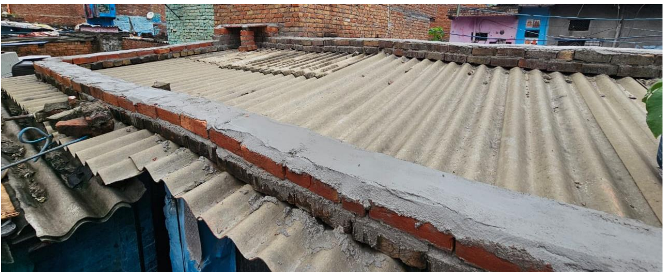
Figure 4.1: Parapet wall after repair works
