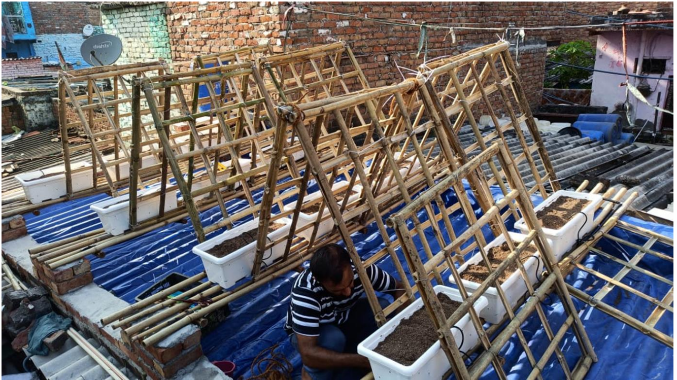
Figure 4.13: Assembling Of Bamboo Trellises
