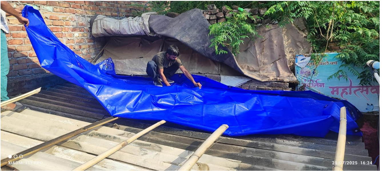
Figure 6.4: Placing Of Silpaulin Above Roof
