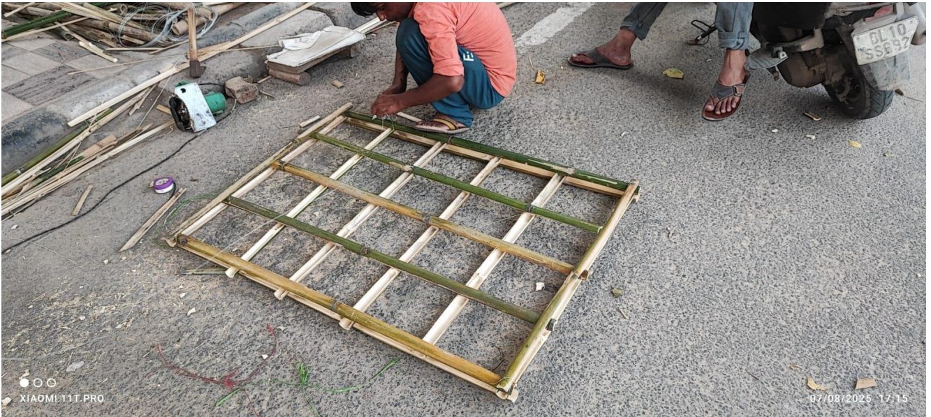
Figure 4.5: Fabrication of Bamboo Frame for Trellis
