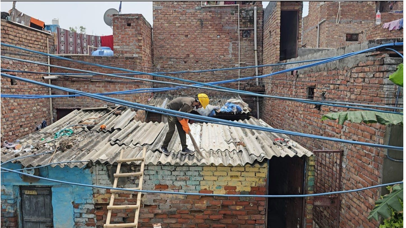
Figure 5.1: Cleaning Of Roof
