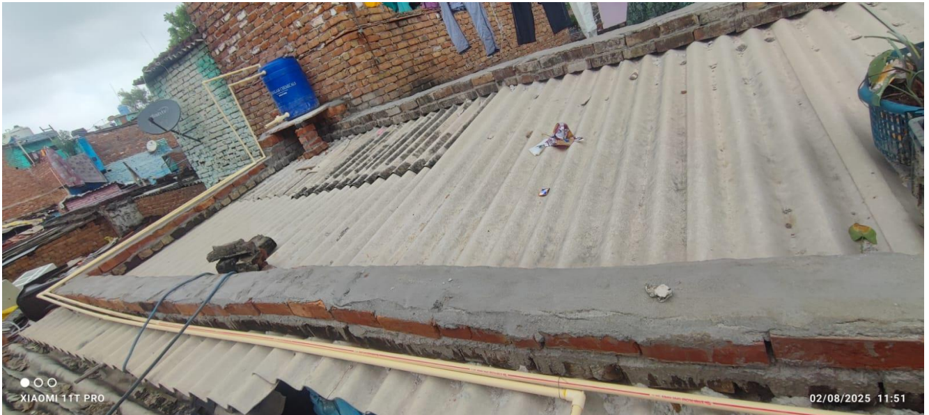
Figure 4.3: Over Head Tank After Installation
