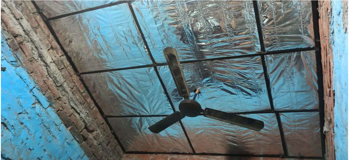
Fig 37.2.5-7 : Metal support framework with panels in place with no gap in the ends
