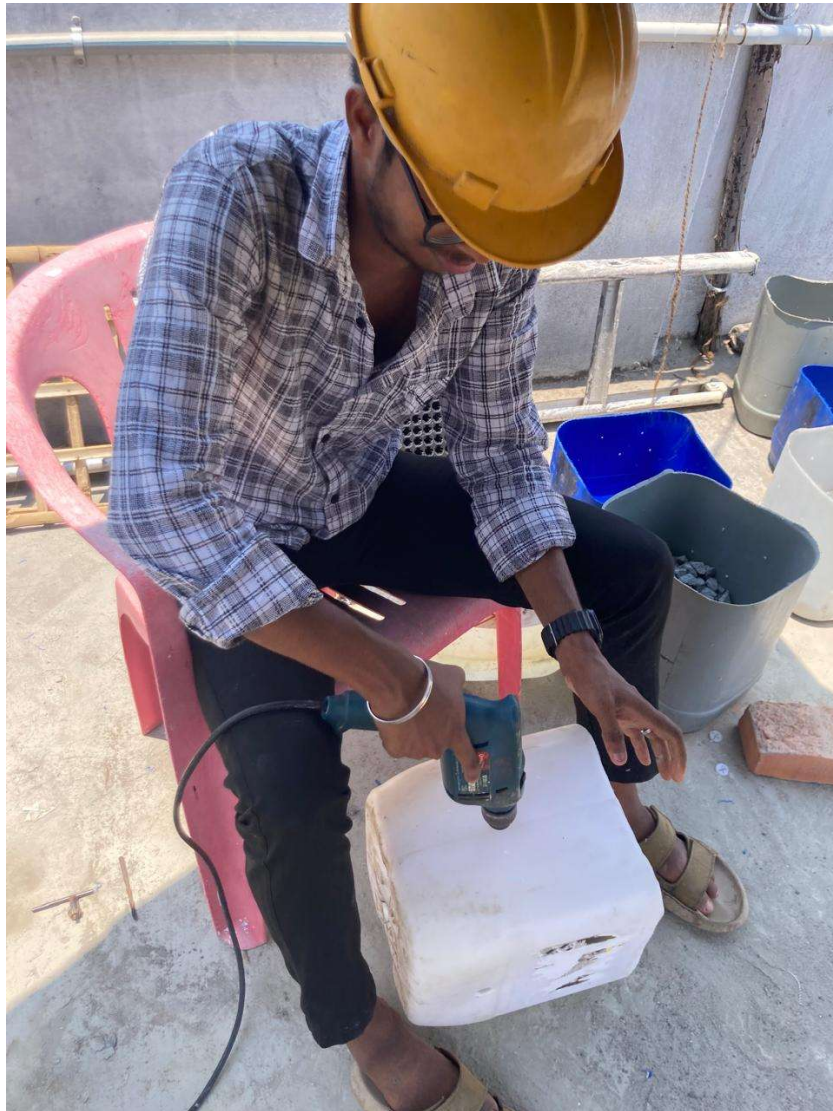
Fig 37.4.2-5 : Drainage hole making on pot
