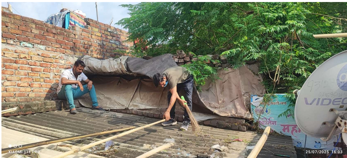
Fig 37.6.1-1 : Cleaning Of Roof
