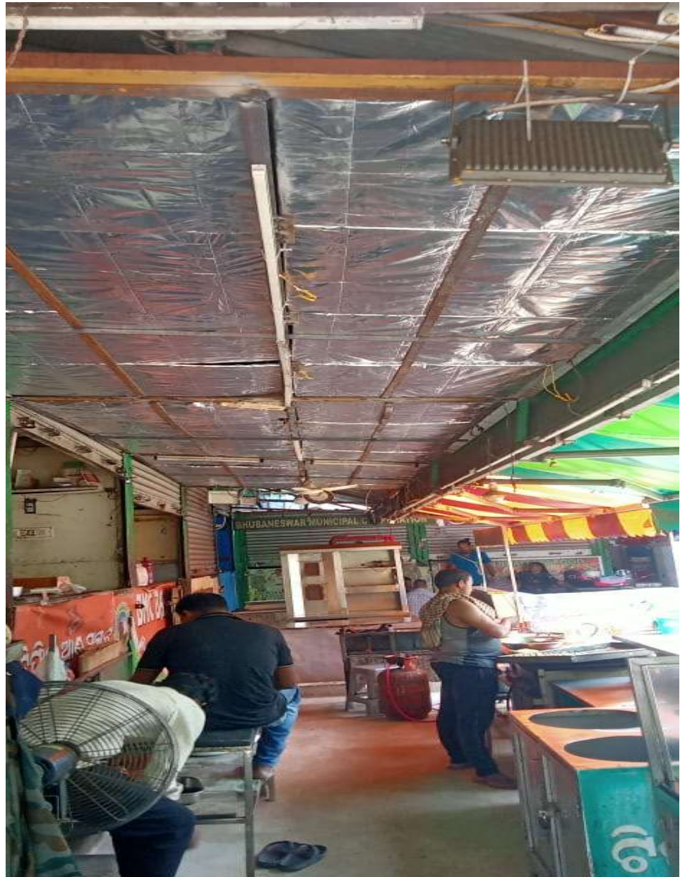
Fig 22.1.2.7-2 : Biomass Panel Installation
