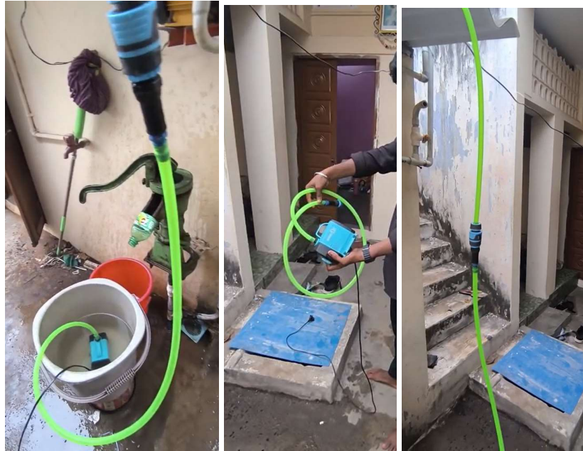
Fig 37.4.2-16 : Submersible installation along with hose pipe
