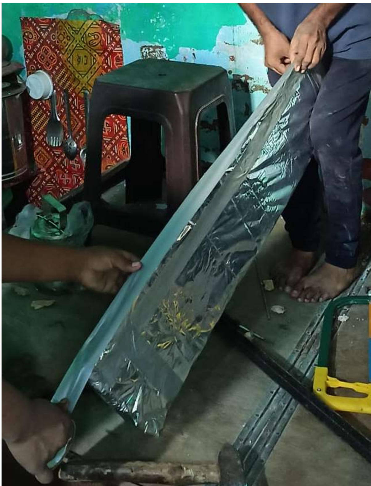
Fig 37.2.5-6 : Tape the cut end with aluminium tape
