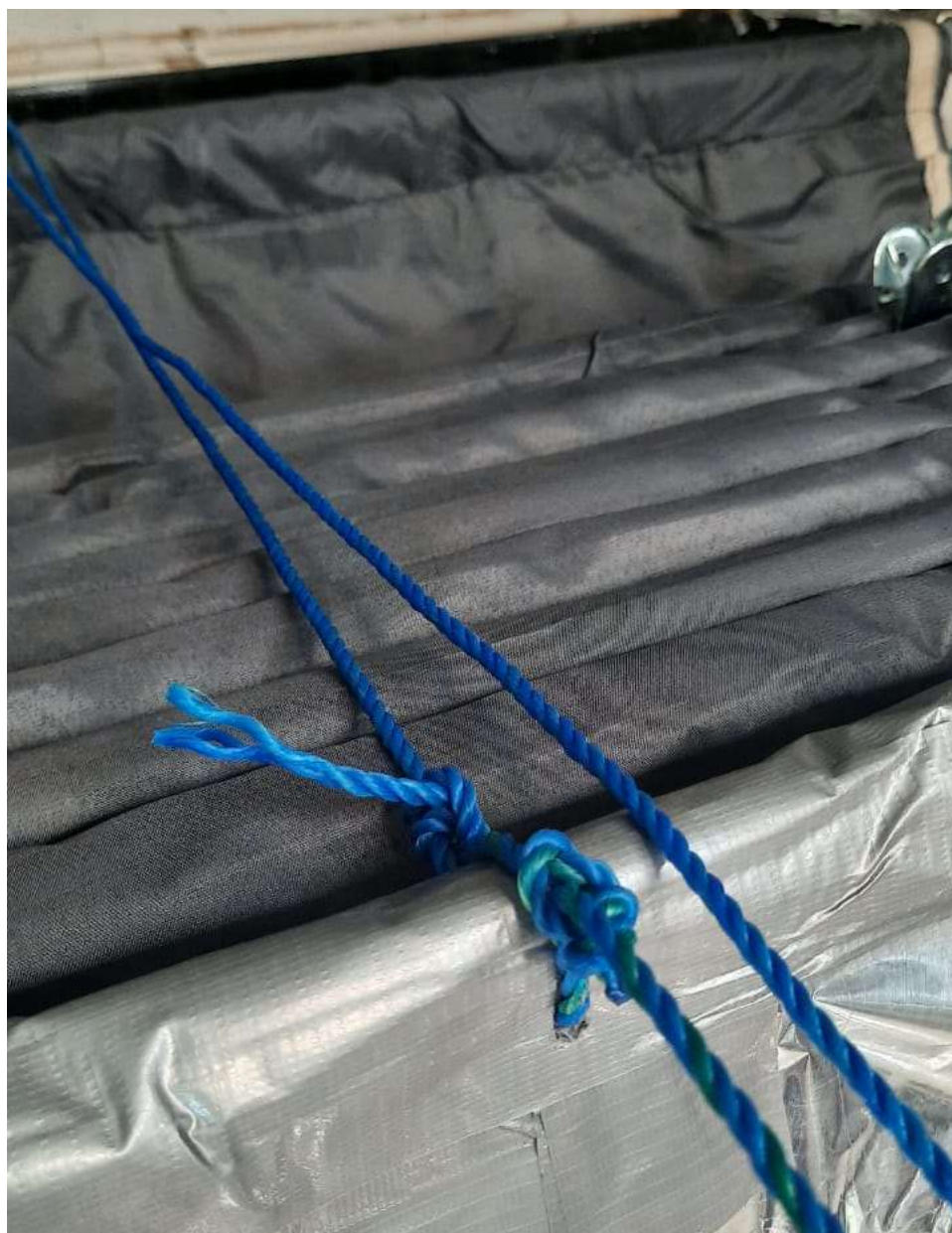
Fig 37.1.3-4 : Attaching nylon rope to the front end pipe of the fractal
