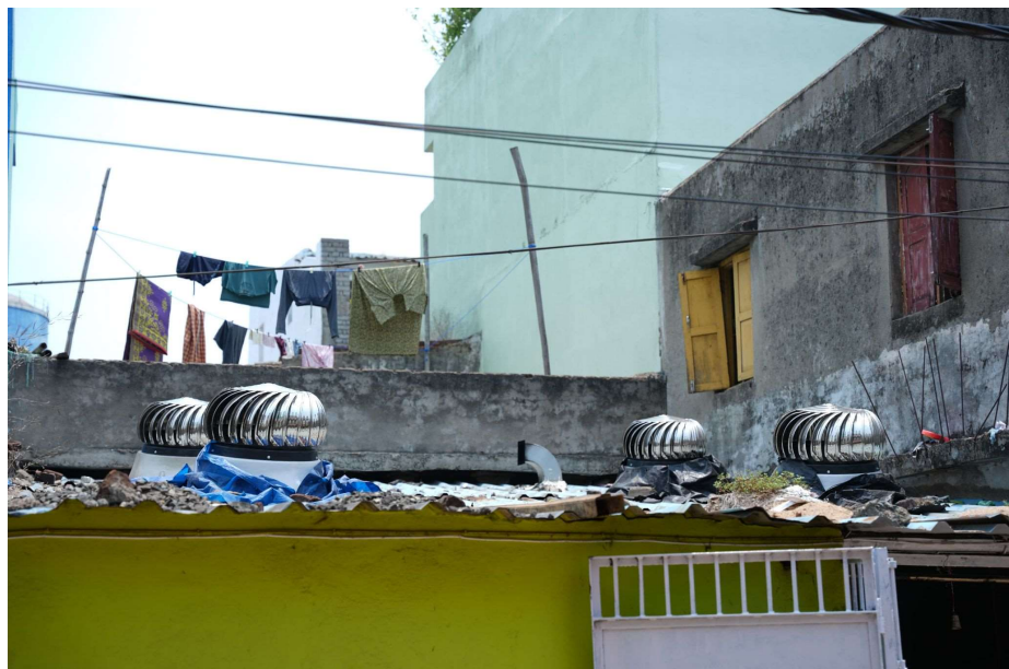
Fig 22.1.1.16-1 : Turbo Ventilator Installation at Baking Space (Outside View)
