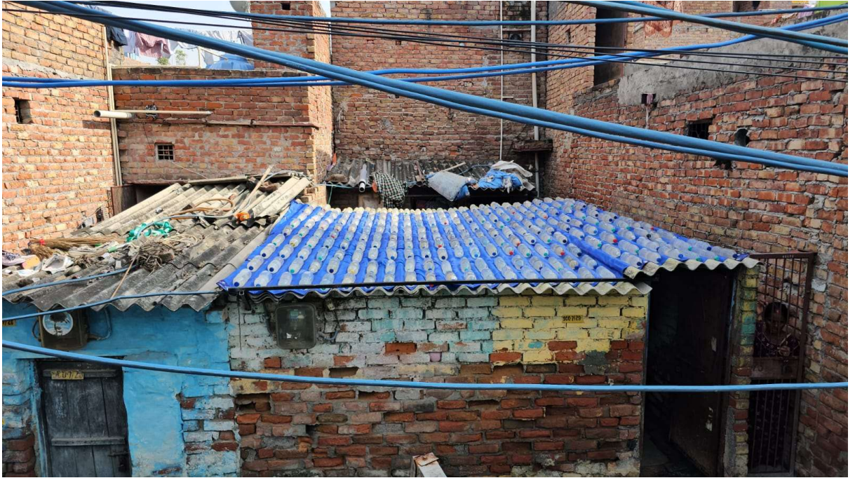
Fig 37.5.3-8 : Final View After MS Strip Installation
