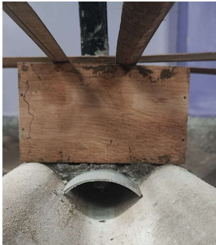
Fig 37.7.2-8 : Casting the support with drip line
