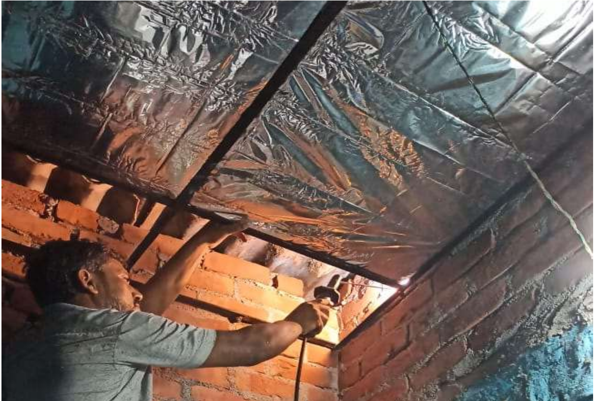
Fig 37.2.5-3: MS support frame in a single plane
