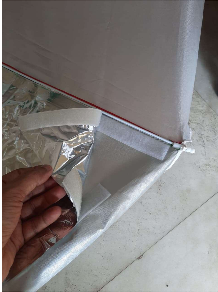
Fig 35.8.1-7 : Attaching of Velcro Strips
