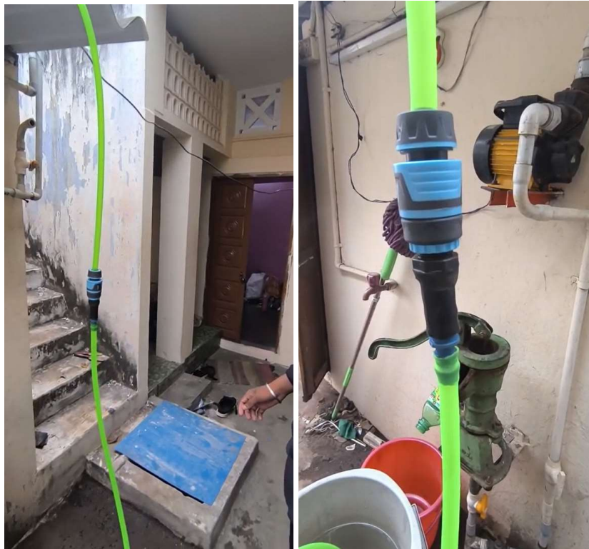
Fig 35.3.4-3 : Easy Removable Hose Pipe Connector
