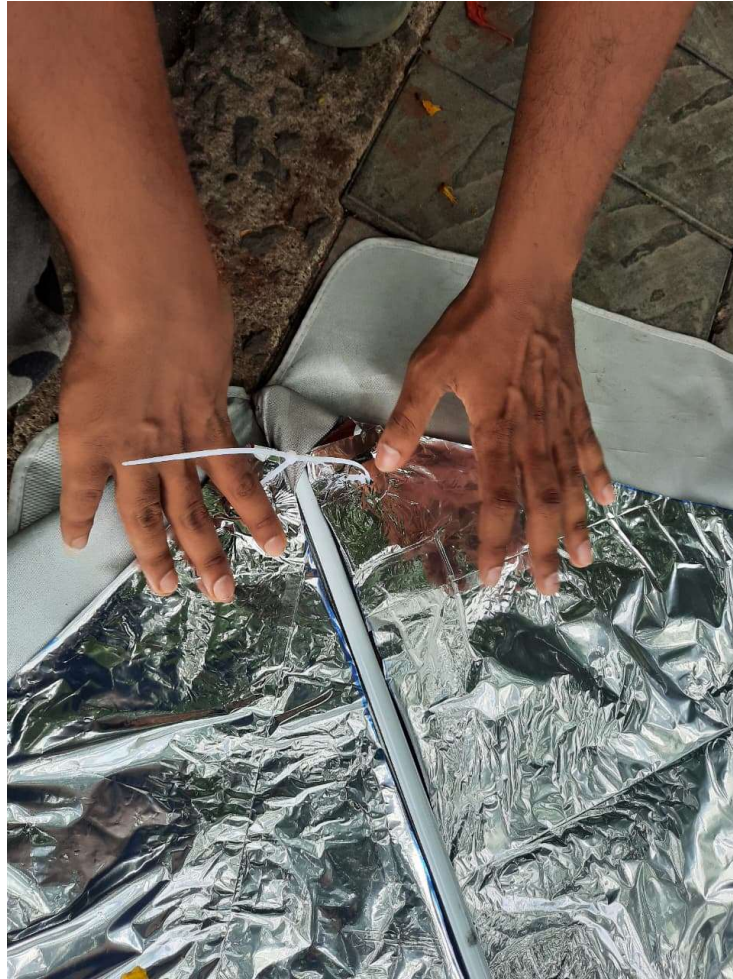
Fig 35.8.1-6 : Securing MLP Panels using Plastic Ties
