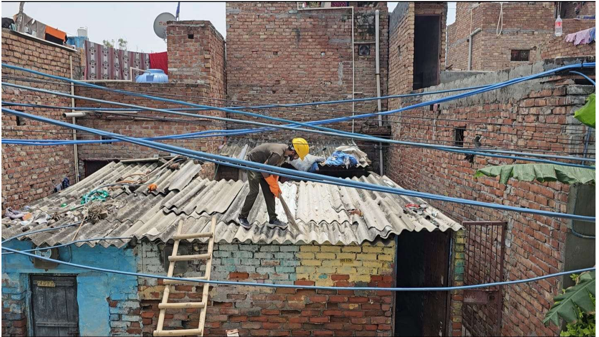
Fig 37.5.1-1 : Cleaning Of Roof
