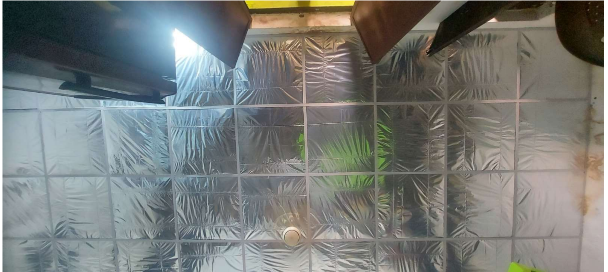
Fig 37.8.3-5 : Aluminum channel framework with all panels in place
