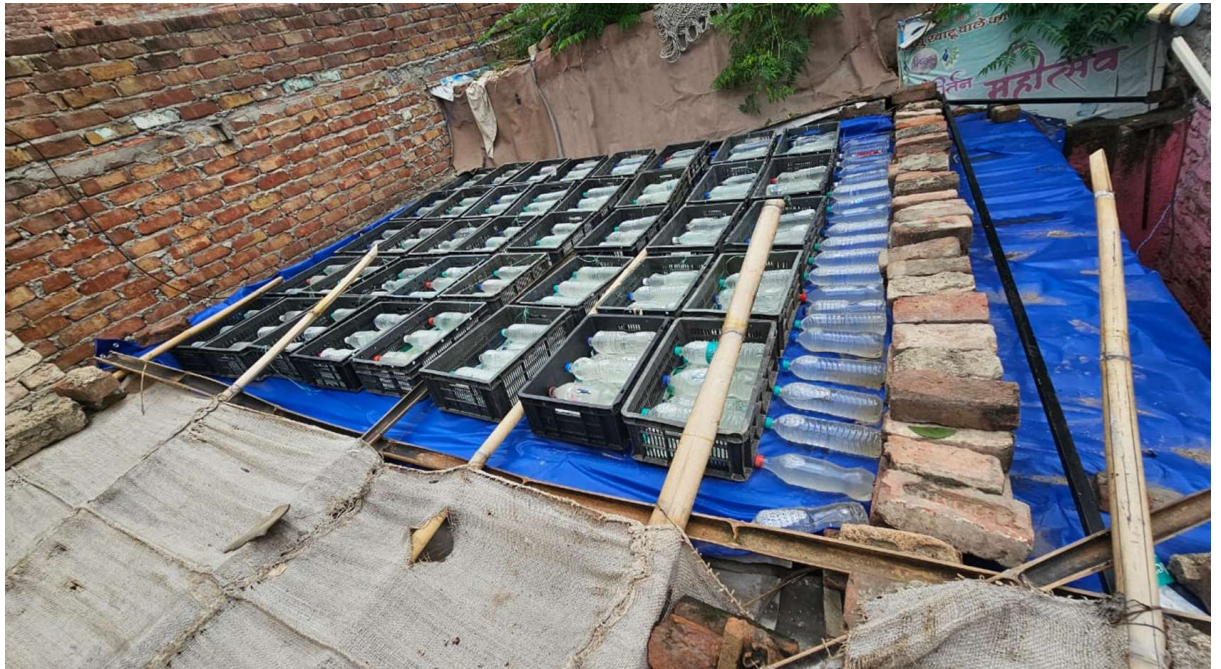
Fig 37.6.3-6 : Final Placement Of Pet Bottle In Crates
