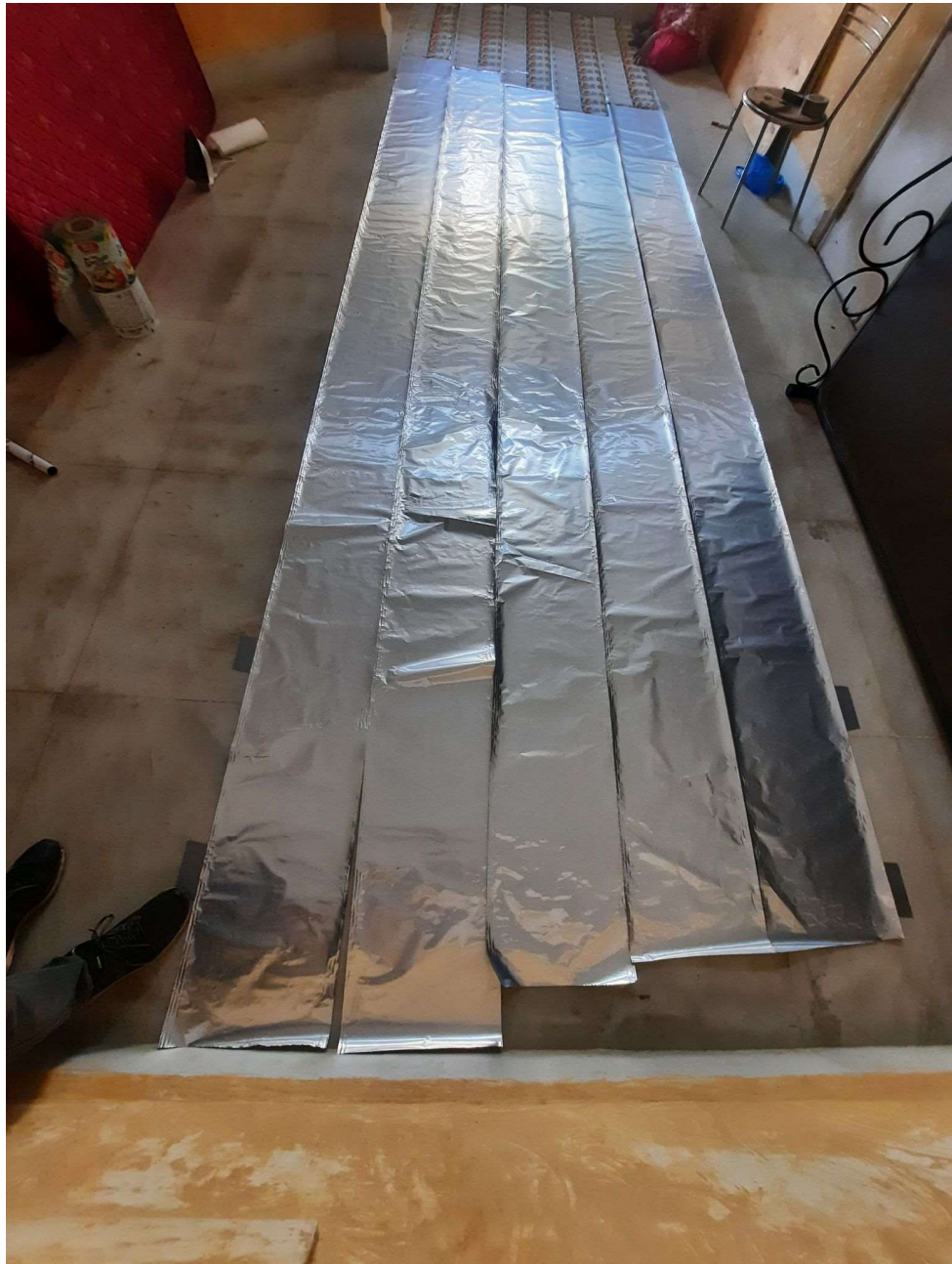
Fig 37.1.2-7 : MLP Roll Strips (1 feet each) placed adjacent to each other to make a 5 feet width panel
