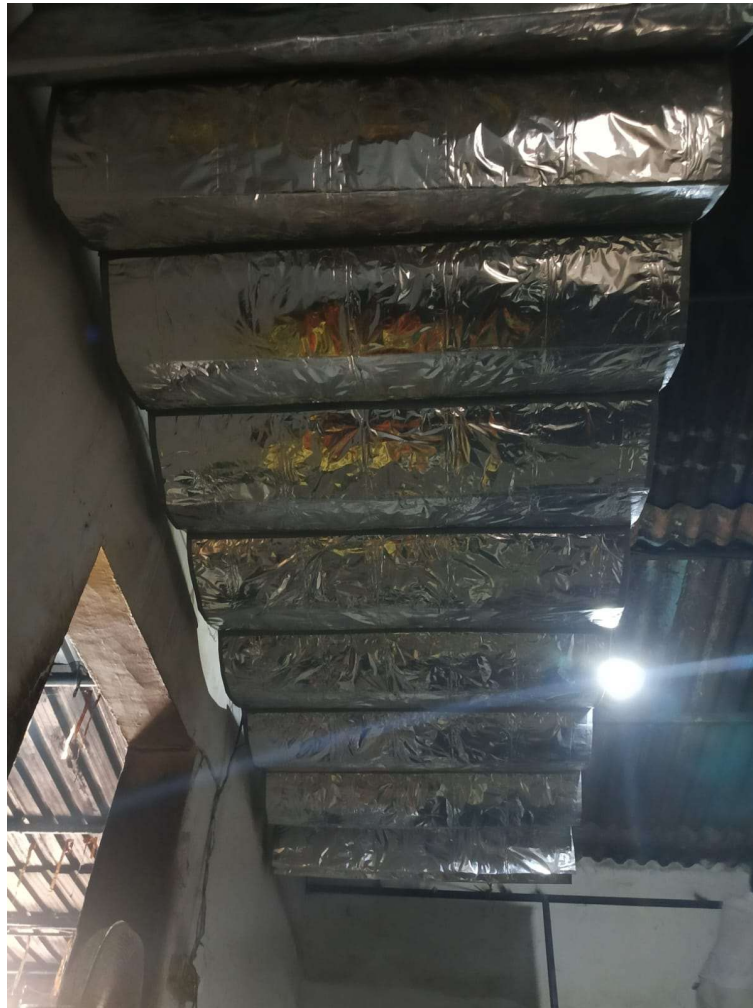
Fig 22.1.1.11-1 : Internal Radiant Barrier Installation
