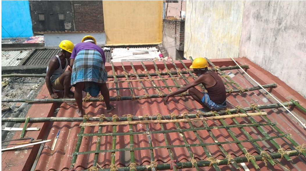
Fig 37.4.2-11 : Bamboo trellis making process
