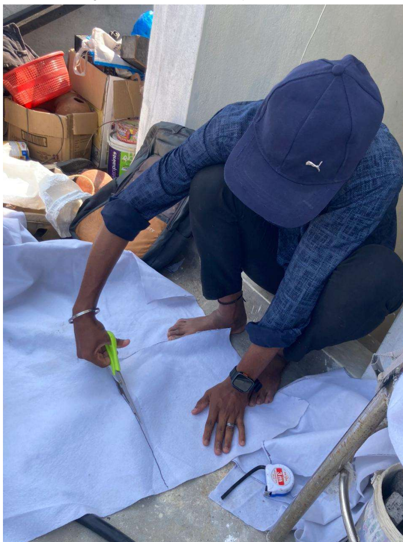
Fig 37.4.2-8 : Cutting geofabric as per the area of pots
