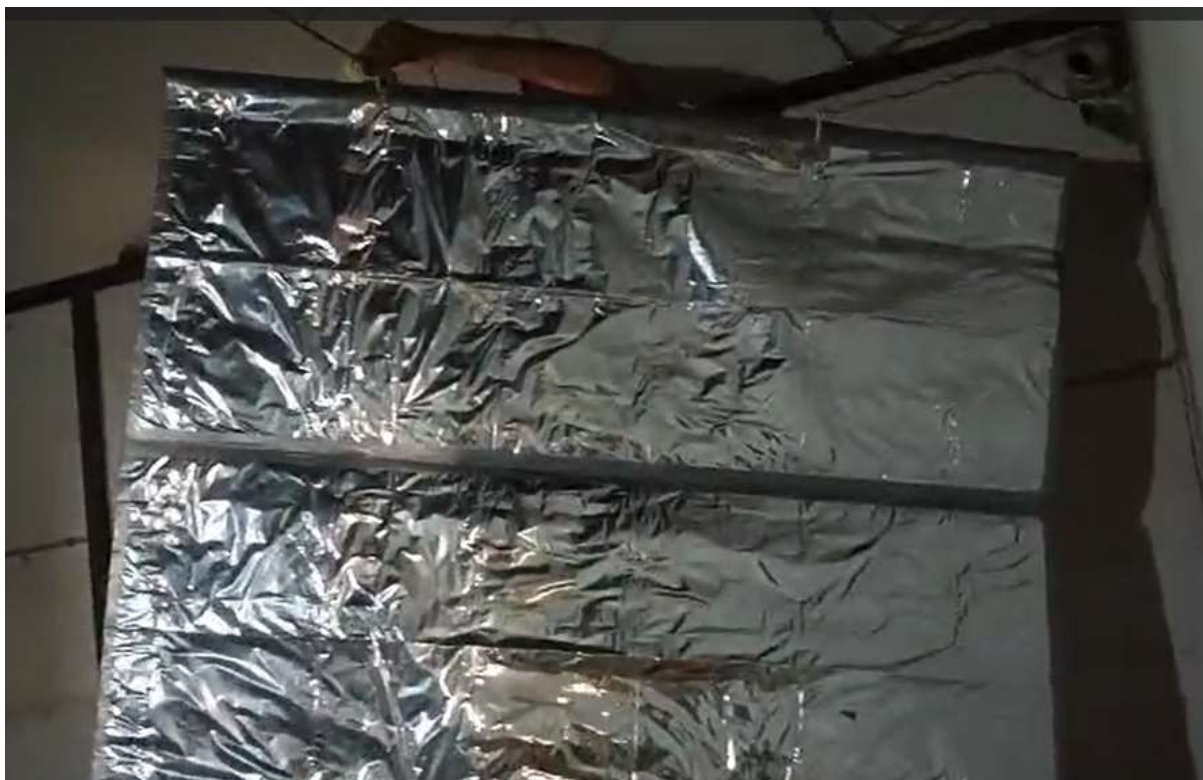
Fig 37.1.3-1 : Hooking of inverted curtain eyelets to the eyelets placed on steel wire.
