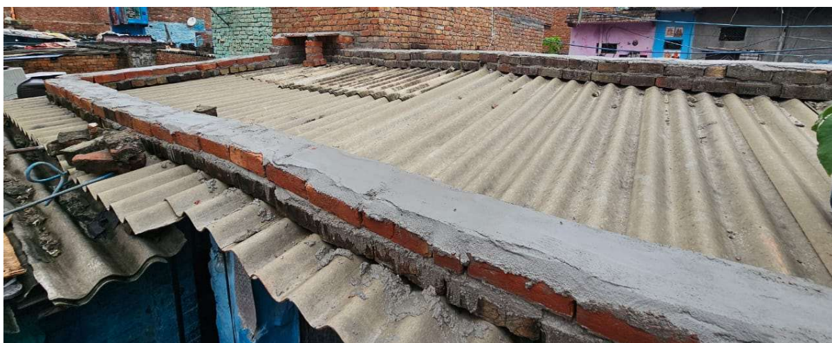
Fig 37.4.1-1 : Parapet wall after repair works
