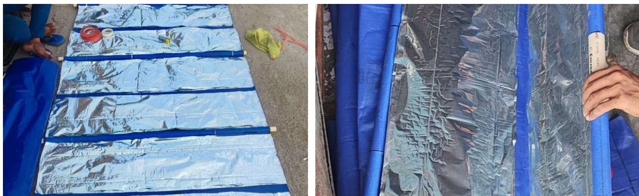
Fig 37.7.2-15 : Inserting intermediary PVC pipes to make the fractal.
