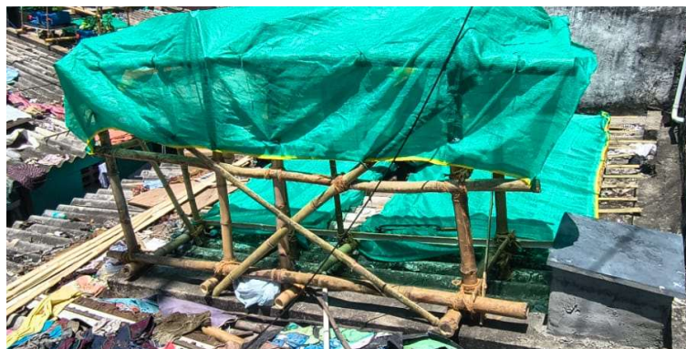
Fig 37.4.2-15 : Scaffolding after finishing all works
