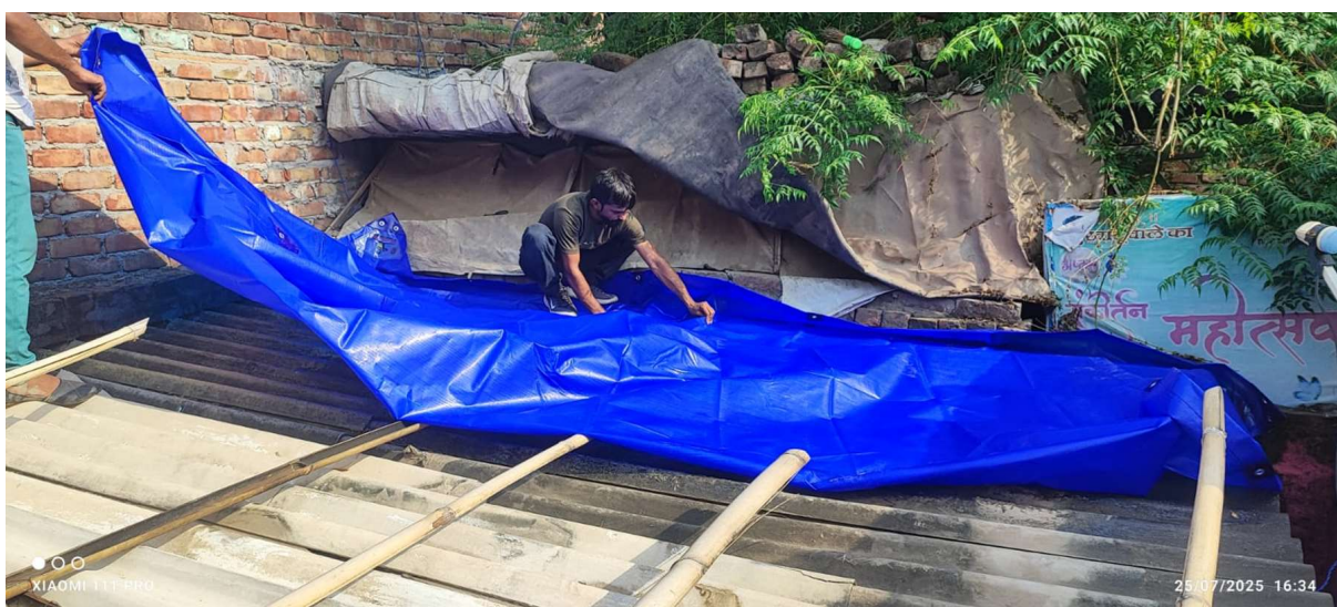
Fig 37.6.3-2 : Placing Of Silpaulin Above Roof
