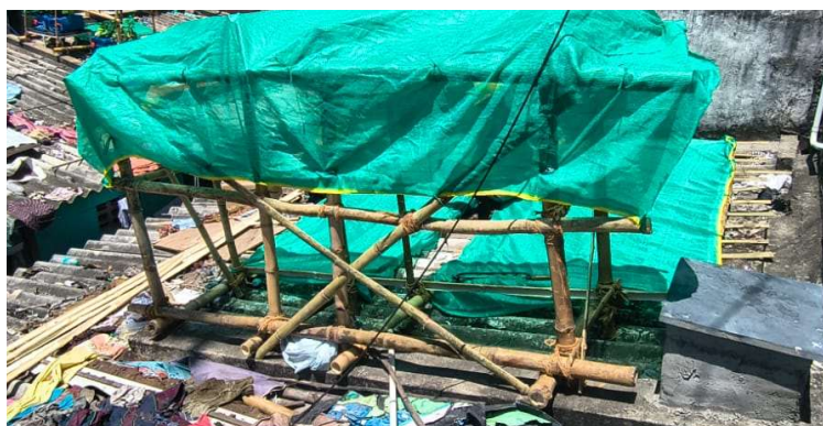
Fig 35.3.3-2 : Scaffolding Structure with Shade Net
