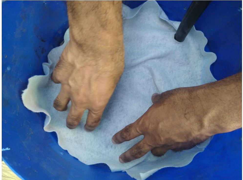
Fig 37.4.2-9 : Place Geofibre on top of concrete chips
