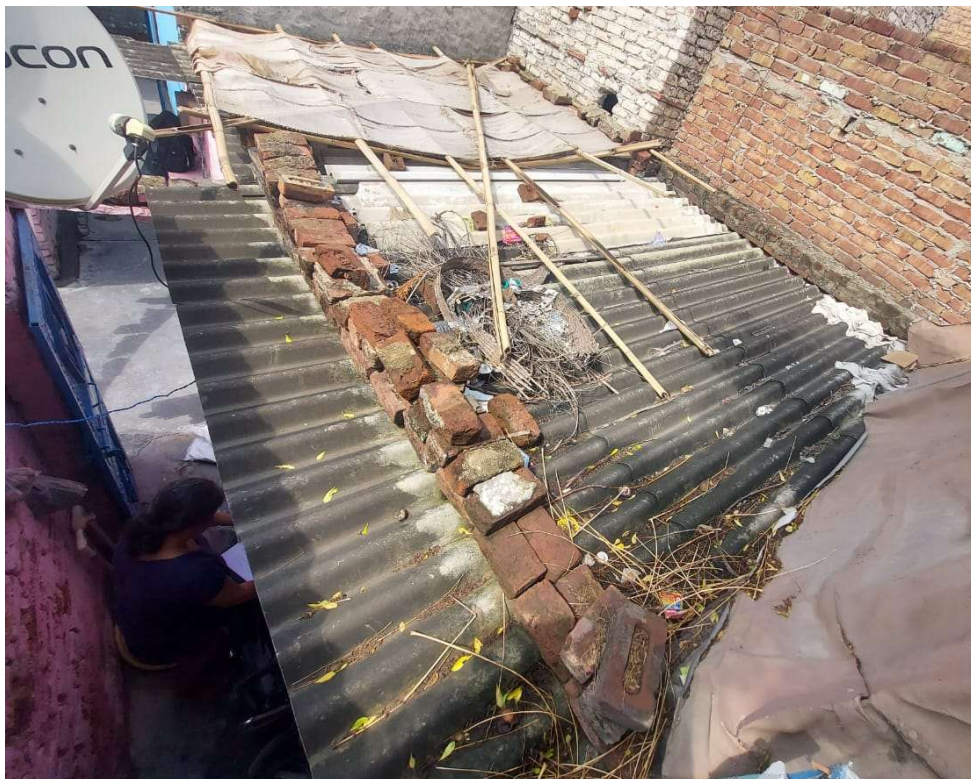
Fig 25.2.1.6-2 : Roof- Top View
