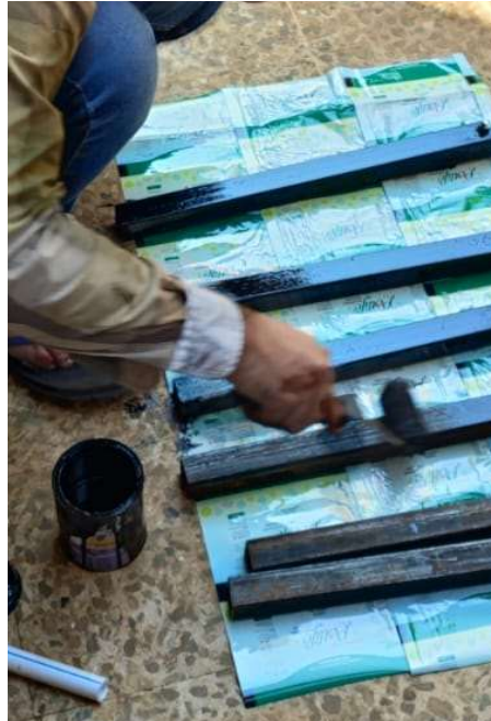
Fig 37.7.2-4 : Painting of Box Sections
