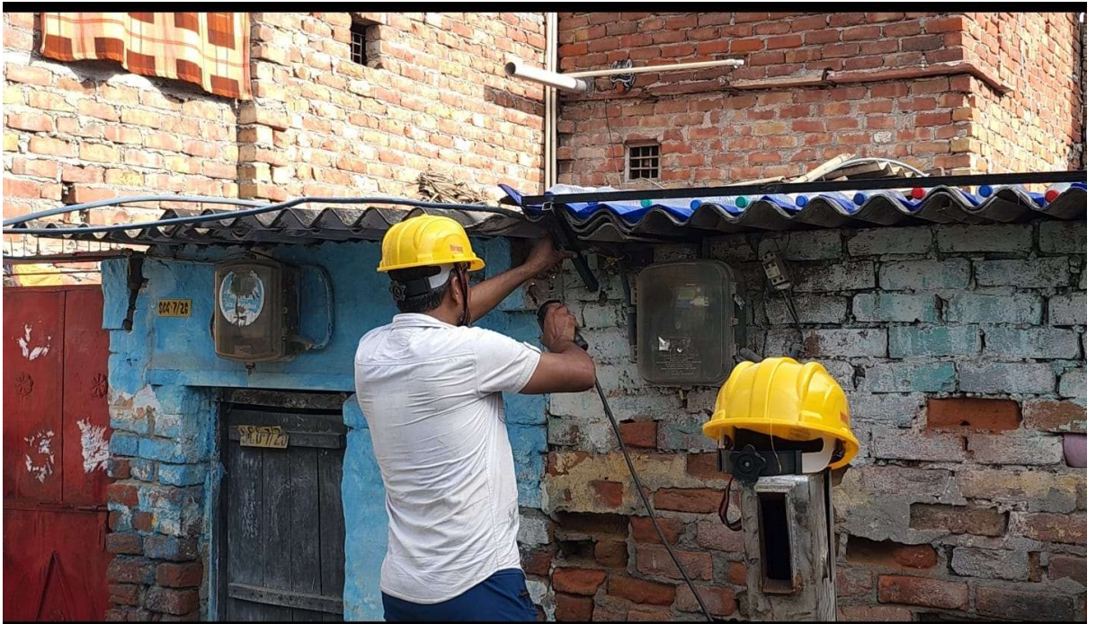
Fig 37.5.3-7 : Securing Of MS Strip Through Welding
