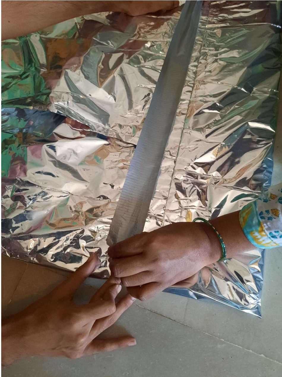
Fig 37.8.2.1.6-1 : Join all the free ends of MLP at the back side of the panel using duct tape.
