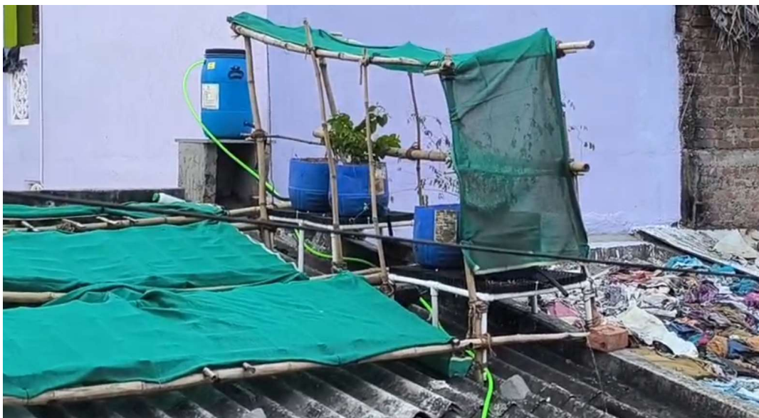
Fig 37.4.2-17 : ½ Hose pipe laid under garden stand connected to over head tank
