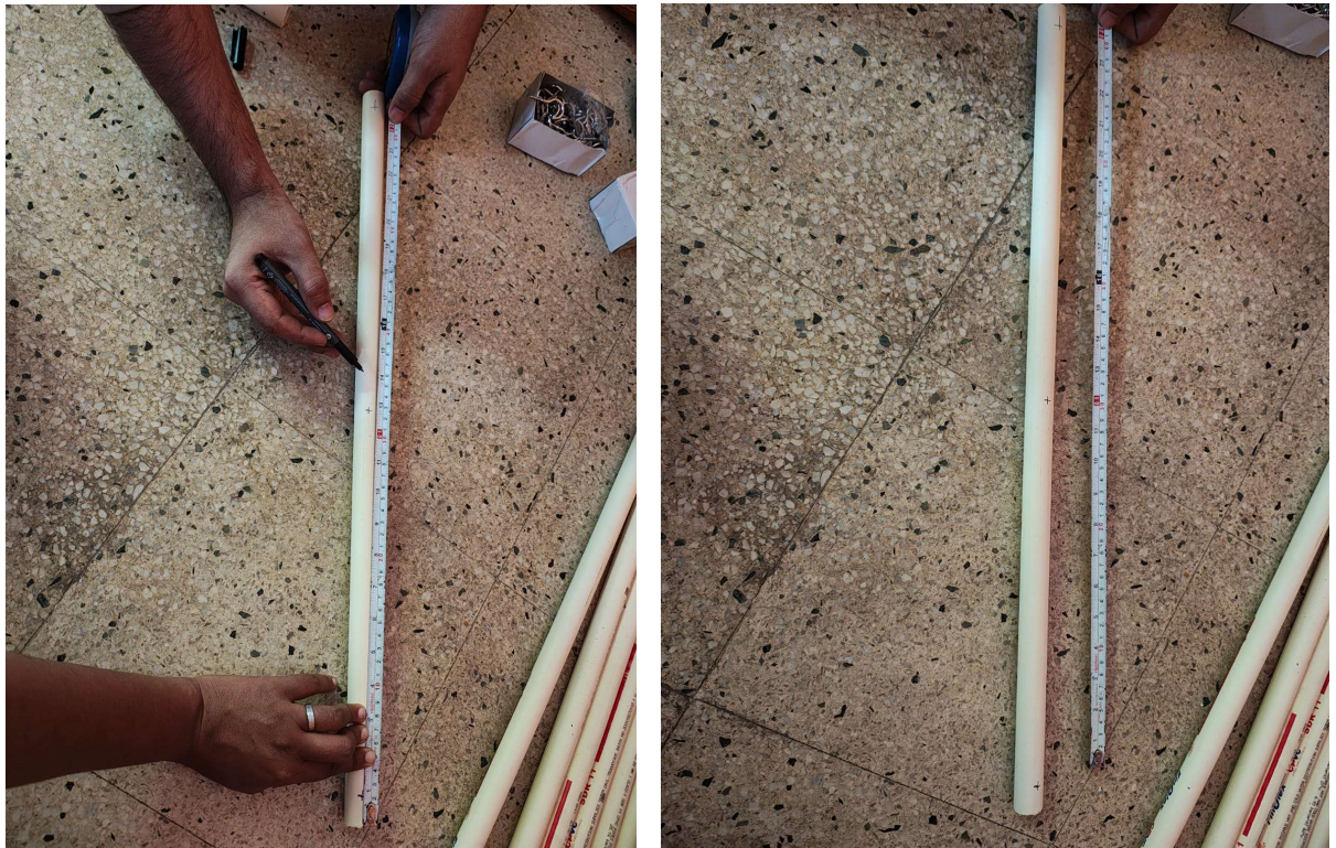
Fig 37.7.2-13 : Marking of points to attach hooks.
