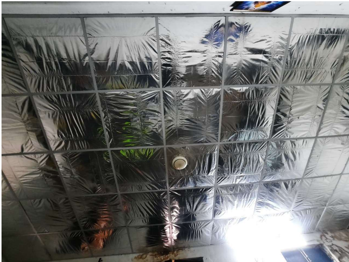
Fig 22.1.6-1 : MLP Static Panel Installation at Office Space
