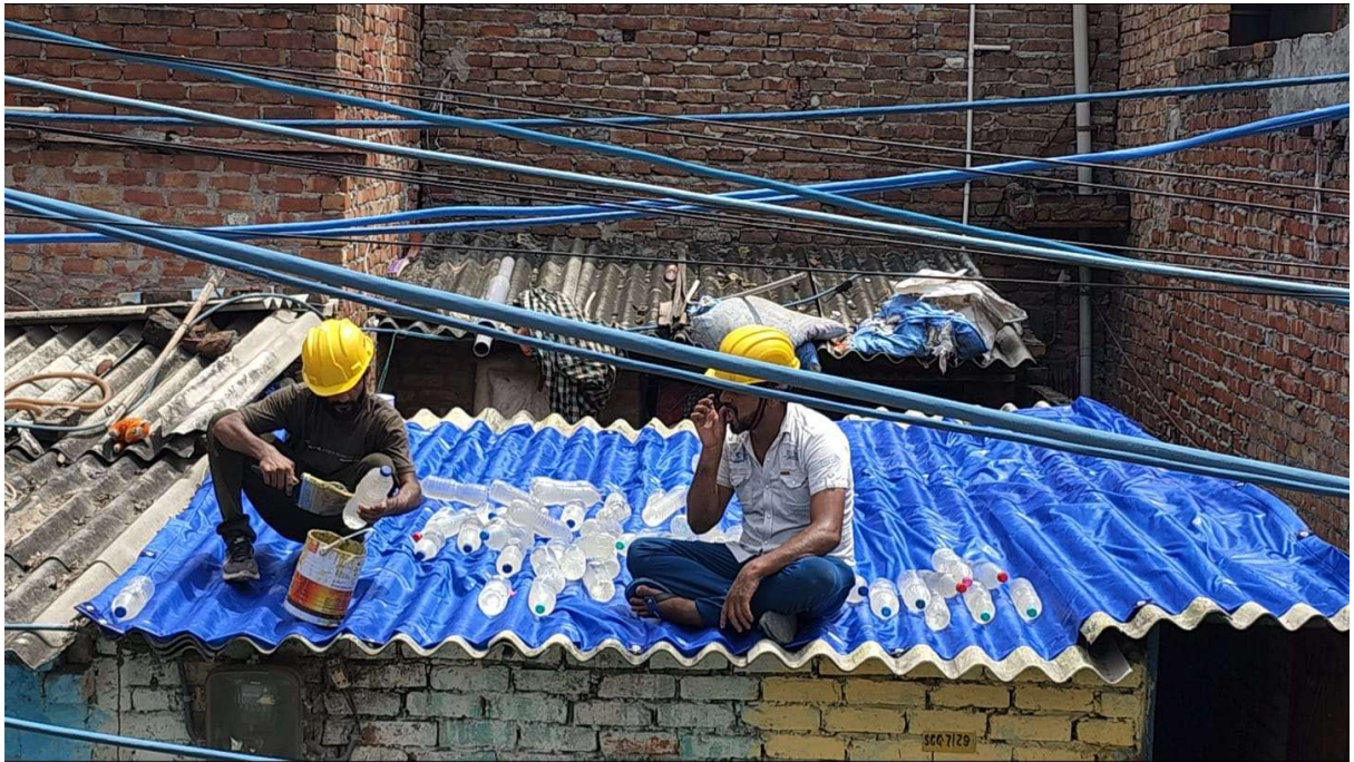
Fig 37.5.3-4 : Application Of Adhesive Along The Bottle Side Which Touches The Roof
