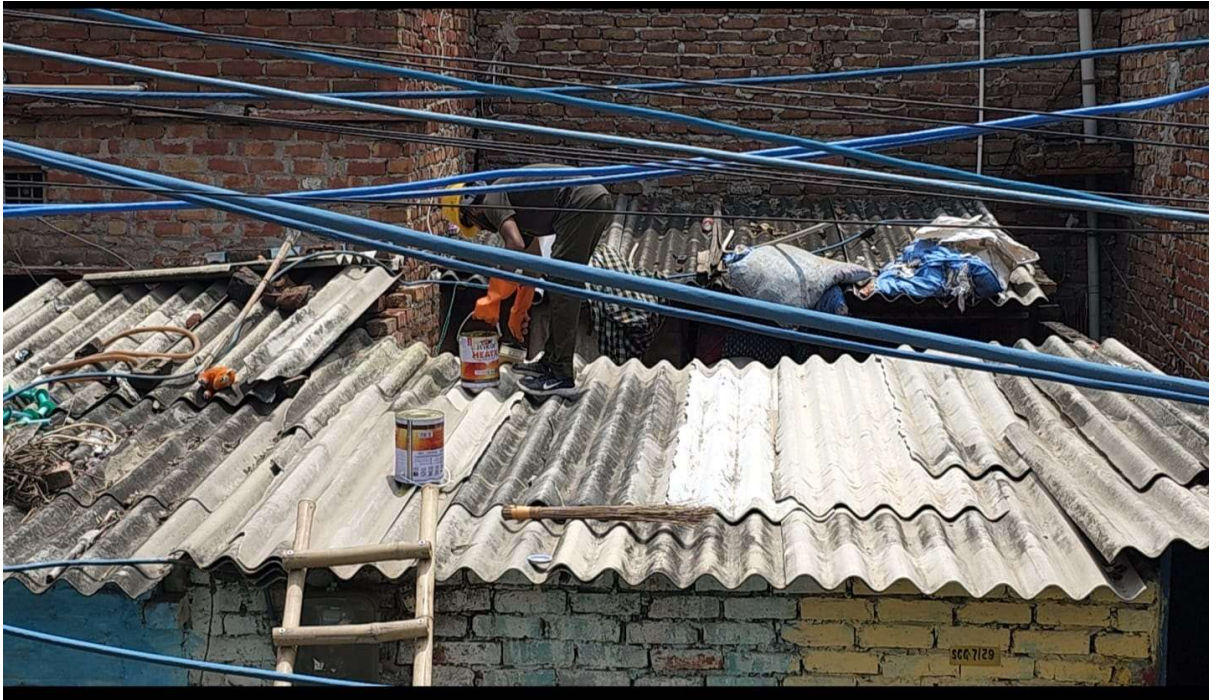
Fig 37.5.3-1 : Applying Of Adhesive Over The Roof
