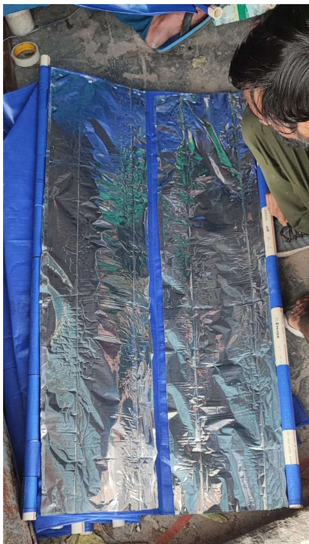
Fig 37.7.2-11 : Attaching MLP to Tarpaulin
