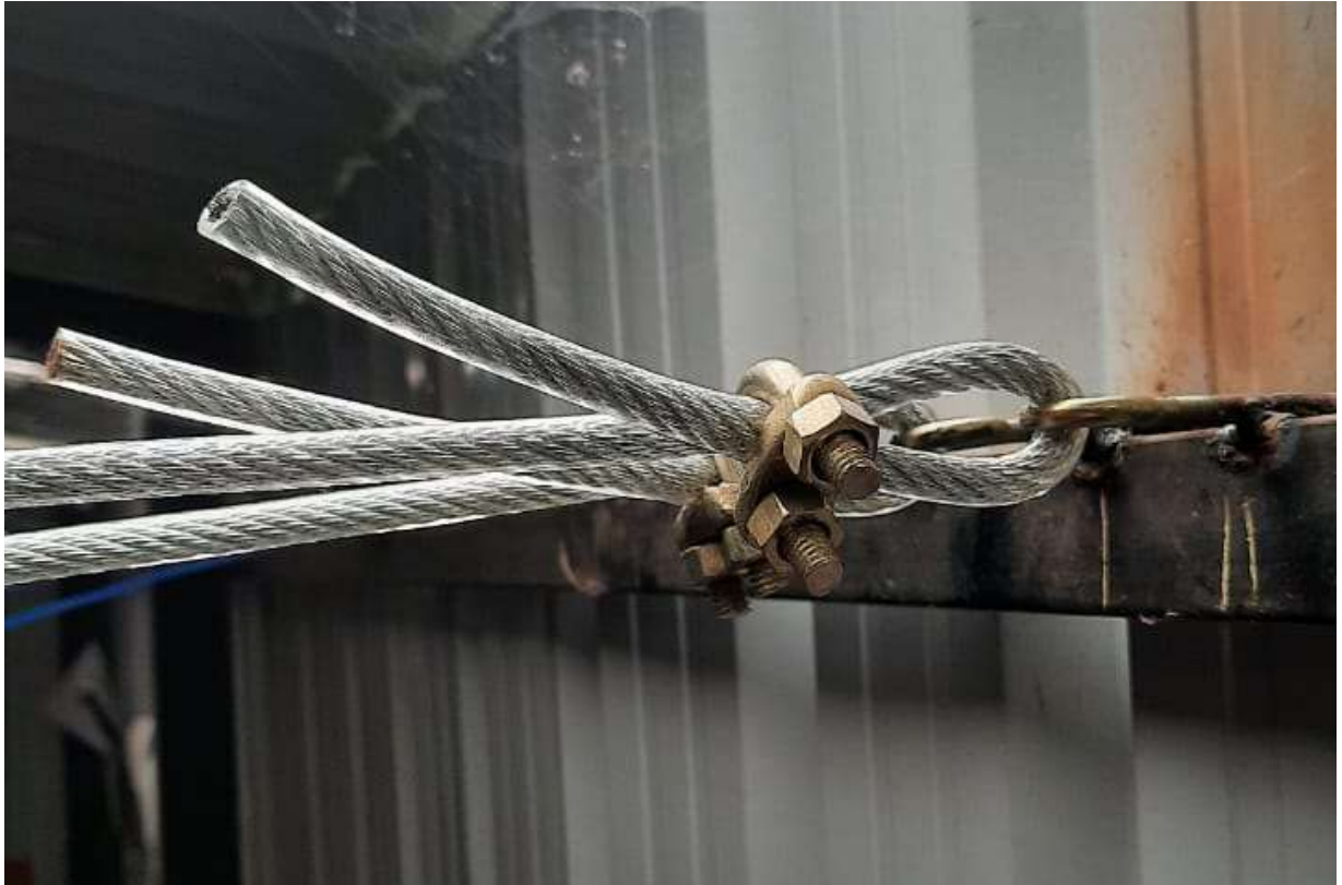
Fig 37.1.2-4 : Establishing wire rope to wall using U-clamps
