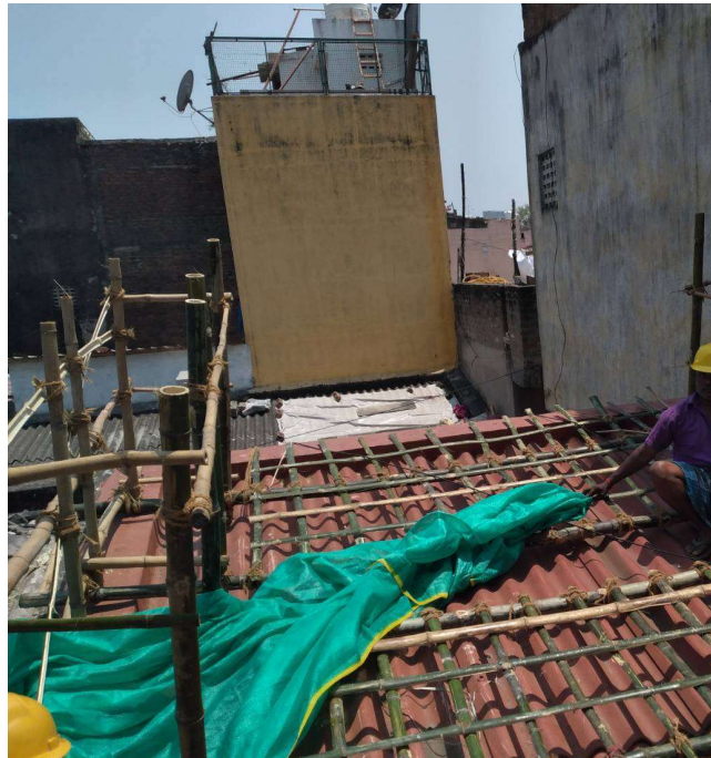
Fig 37.4.2-12 : Green net attaching to the Bamboo trellis
