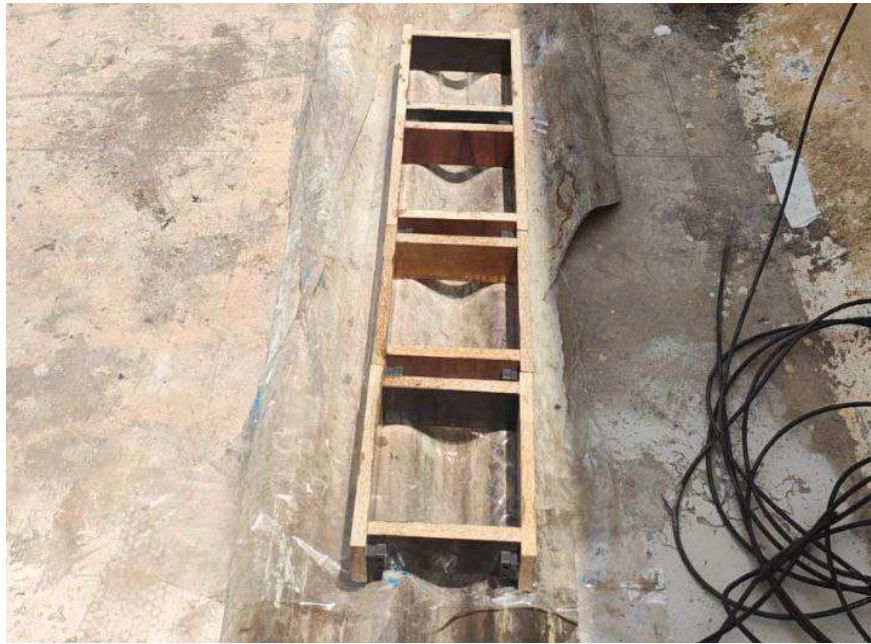
Fig 37.7.2-5 : Placing of moulds on roofing sheet
