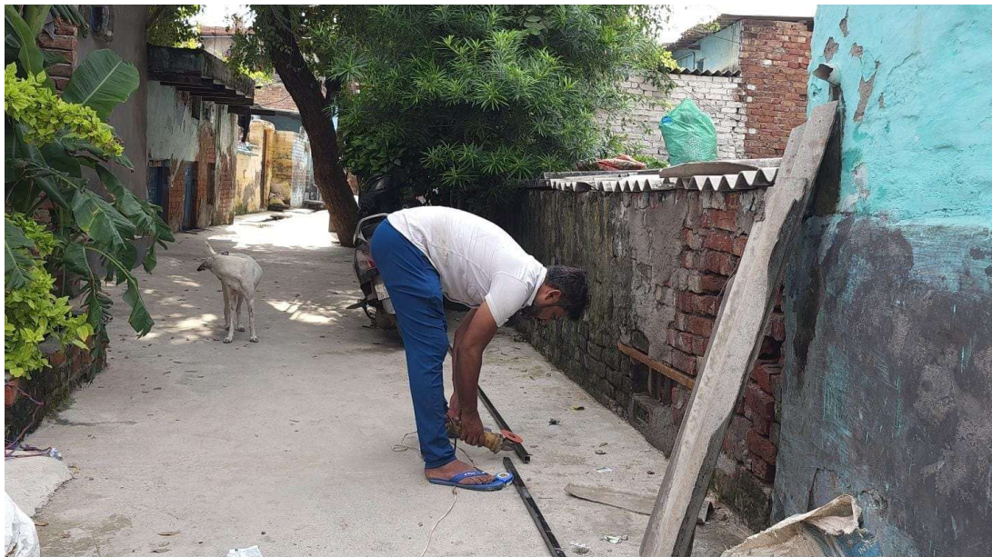
Fig 37.5.2-2 : Cutting Of MS Strip
