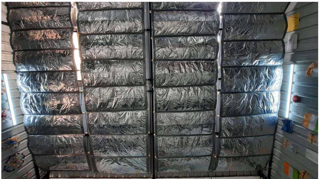
Fig 37.1.3-8 : Fractals (in open position) covering the underside of the Roof.
