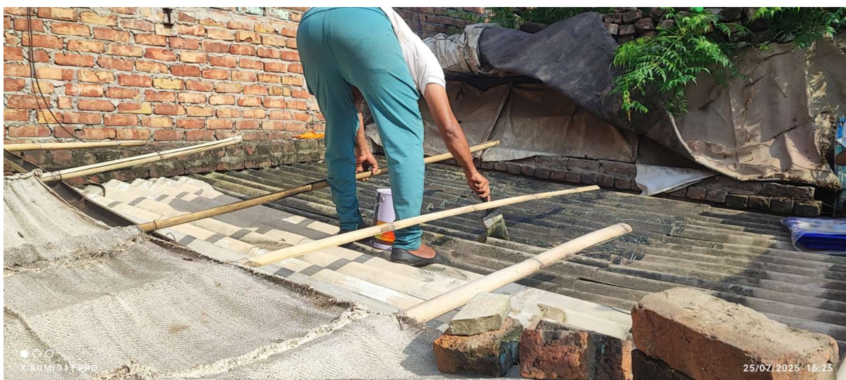
Fig 37.6.3-1 : Applying Of Adhesive Above The Roof
