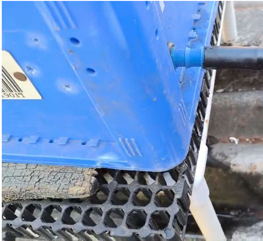
Fig 37.4.2-4 : Washer and connector attached to the pot
