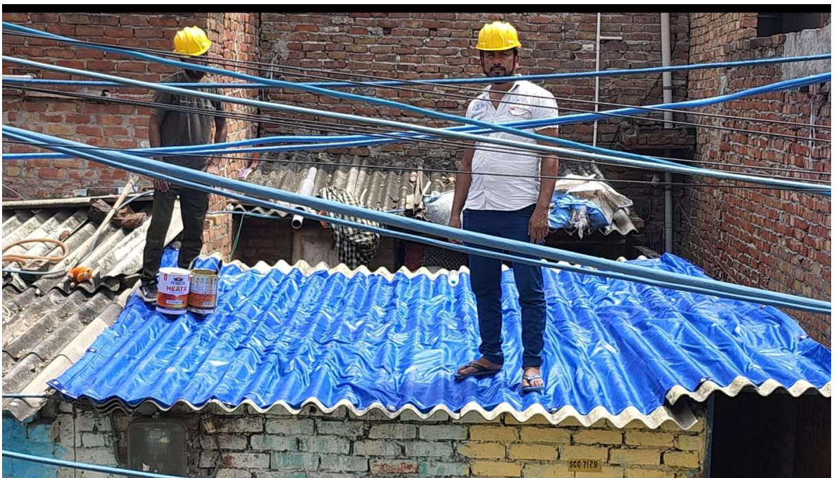
Fig 37.5.3-3 : Final View After Application Of Silpaulin
