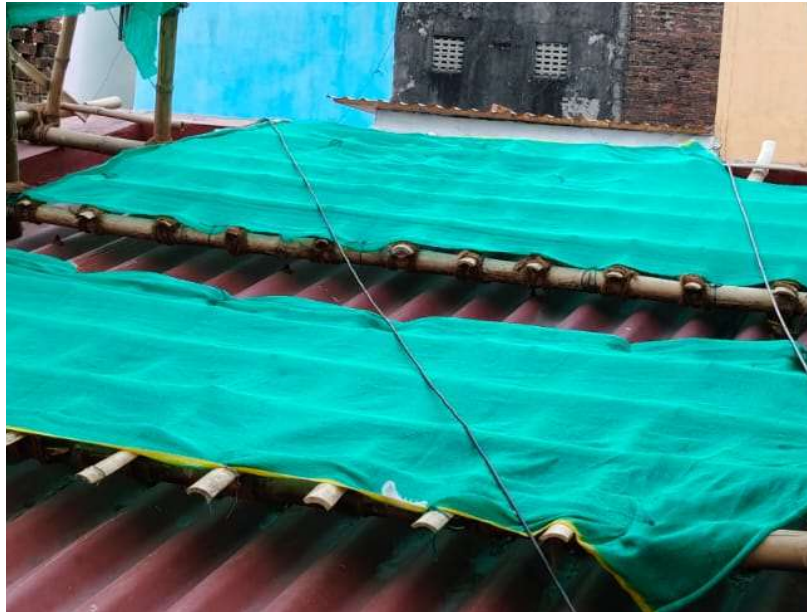
Fig 37.4.2-13 : Trellis after finishing all works
