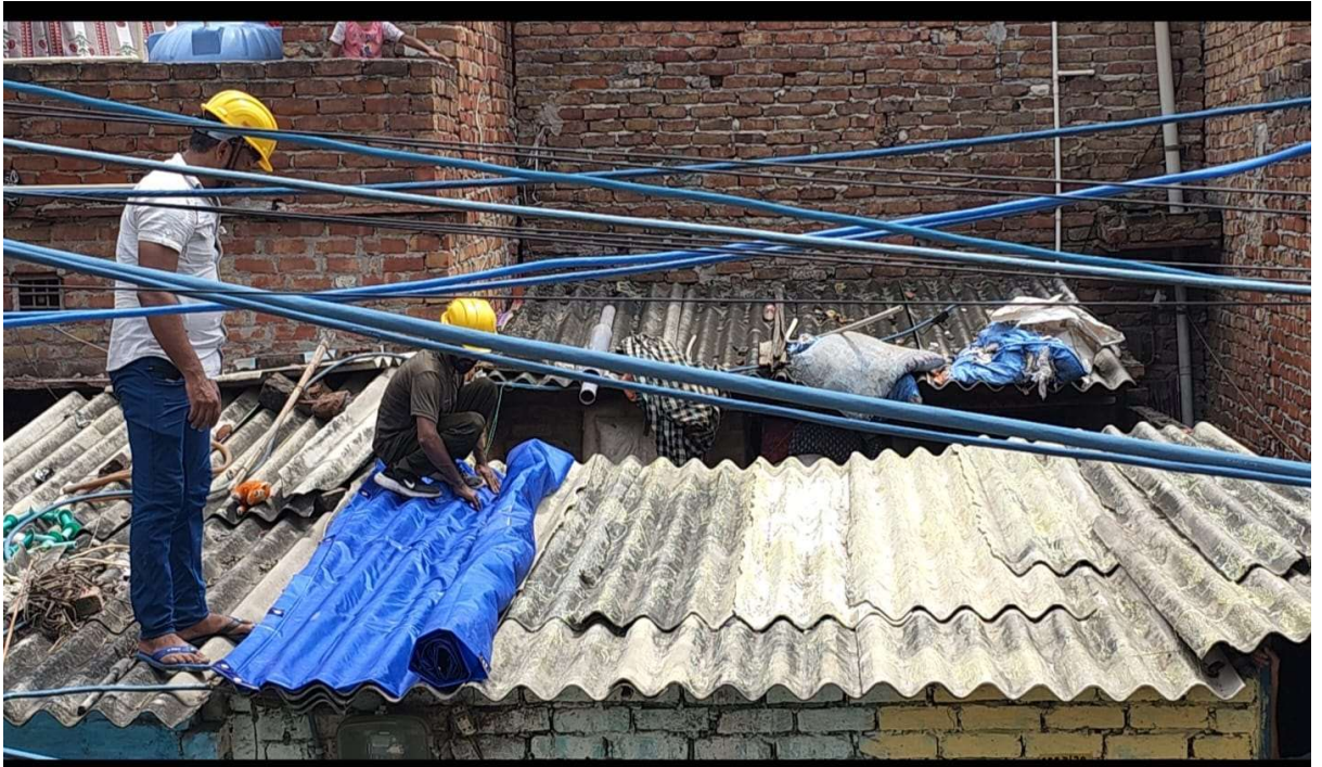
Fig 37.5.3-2 : Sticking Of Silpaulin Across The Roof
