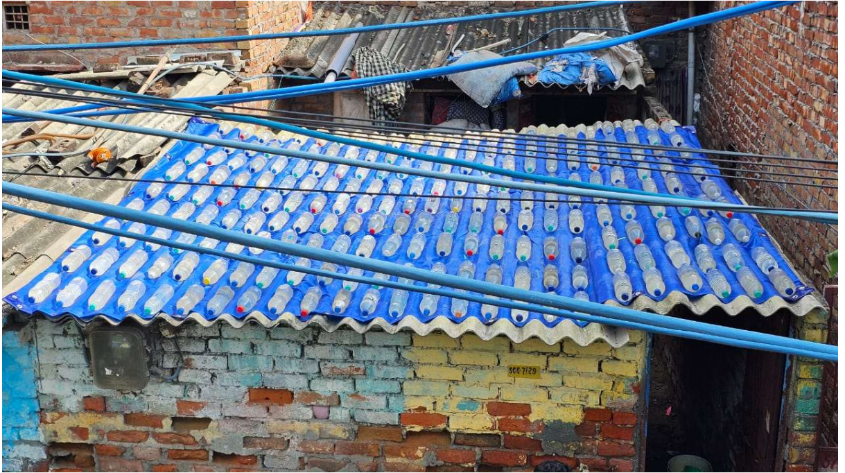
Fig 37.5.3-6 : Final View After Placing Of PET Bottles
