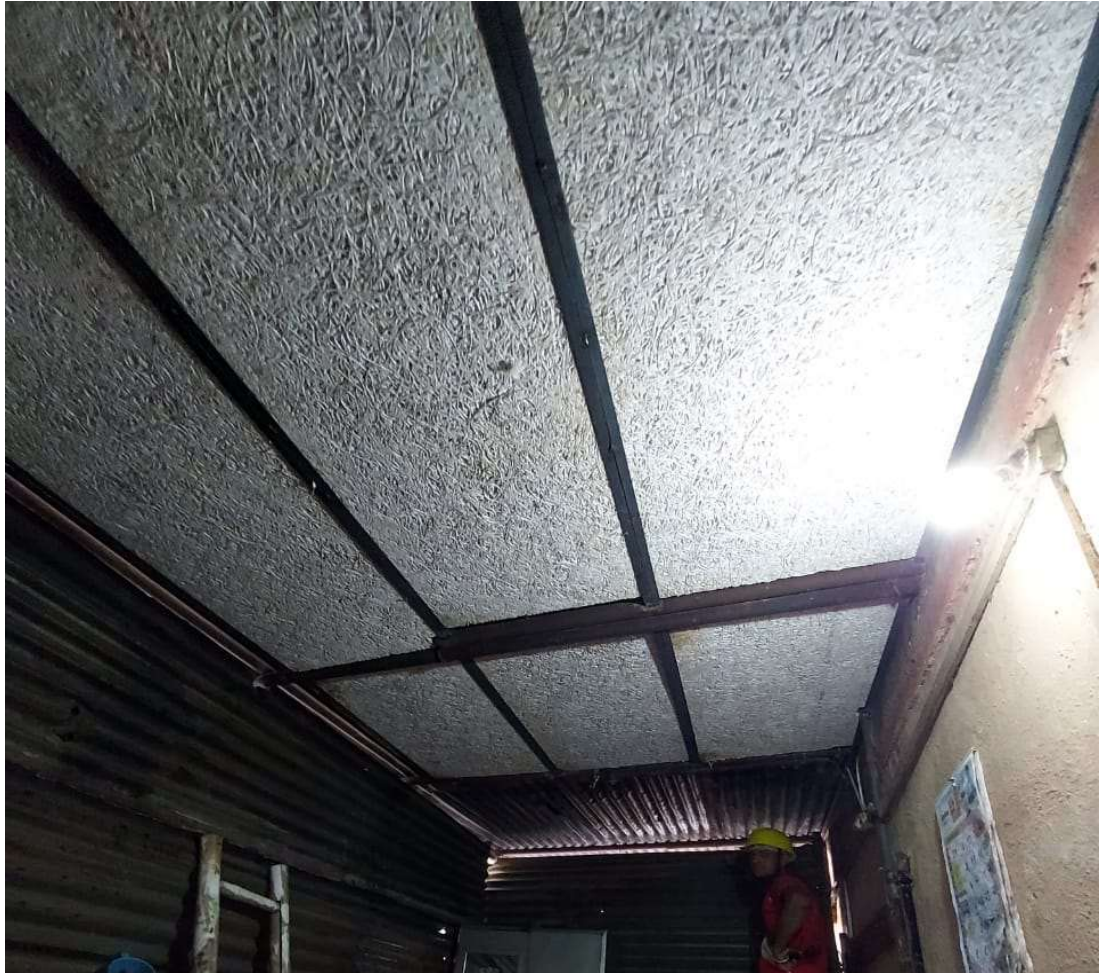
Fig 37.3.2-5 : MS support framework with panels in place
