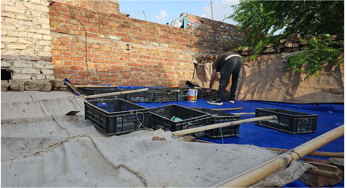
Fig 37.6.3-3 : Placing Of Crates Above Roof
