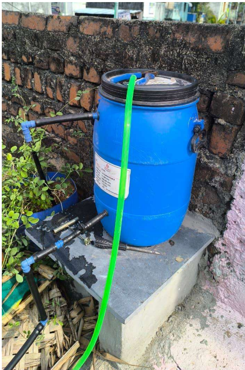
Fig 37.4.1-1.5-1 : Over Head Tank After Installation
