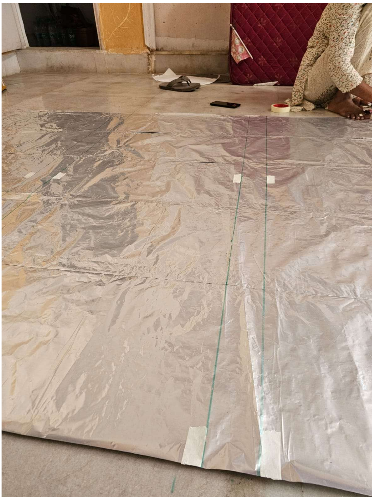
Fig 37.1.2-11 : Placing paper tape for marking 3 inch loop
