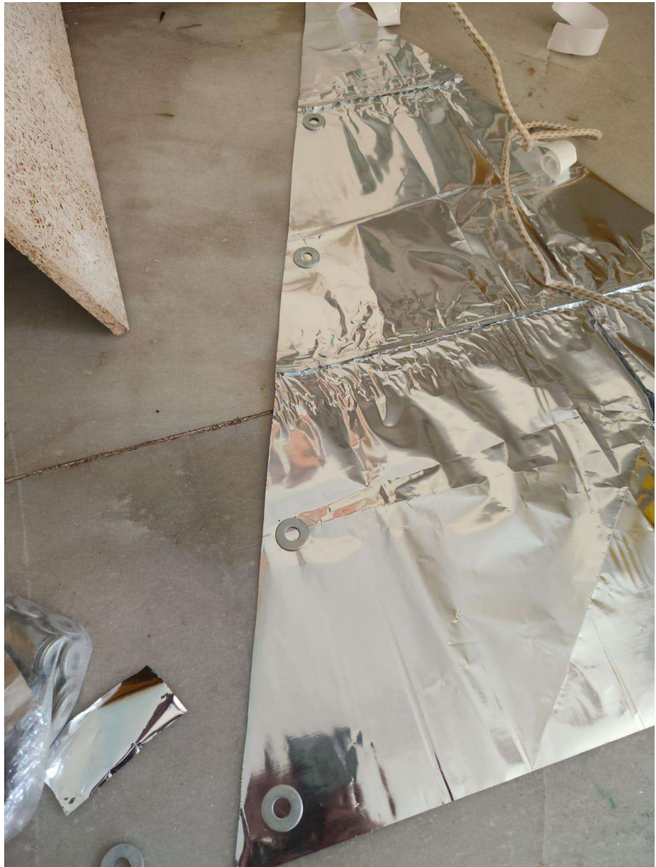
Fig 35.8.1-2 : Placing of SS washers
