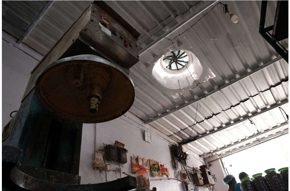
Fig 22.1.1.16-2 : Turbo Ventilator Installation at Baking Space (Inside View)
