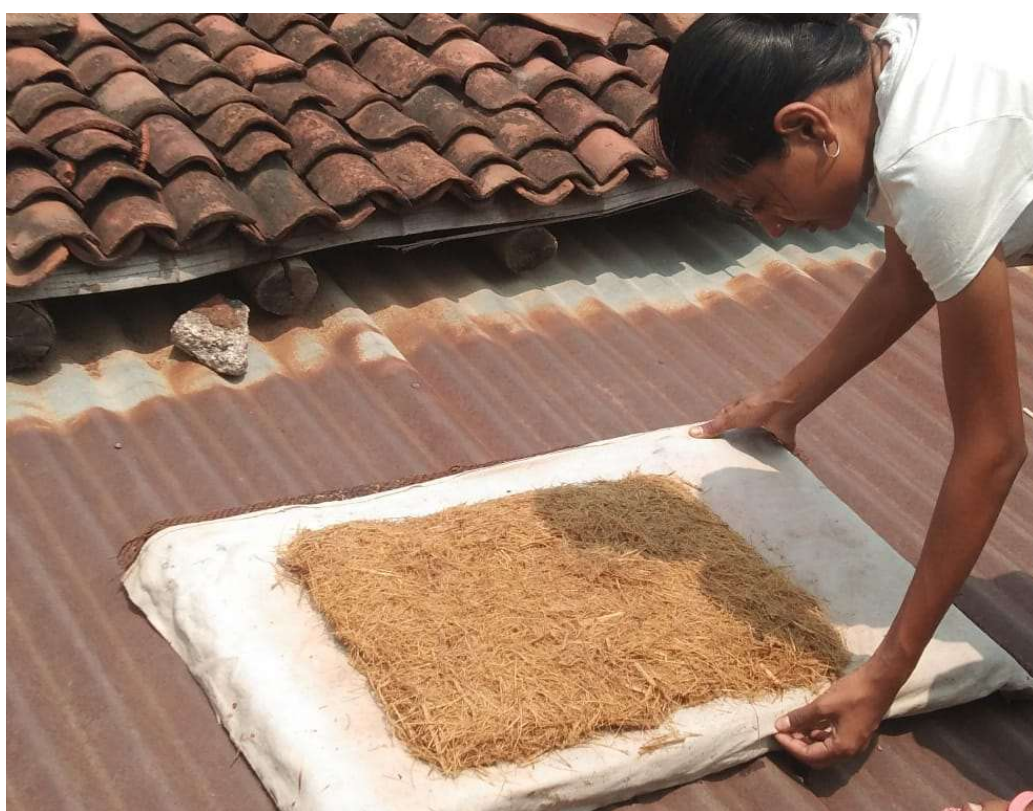
Fig 37.2.2-12: Sun-dry the panels
